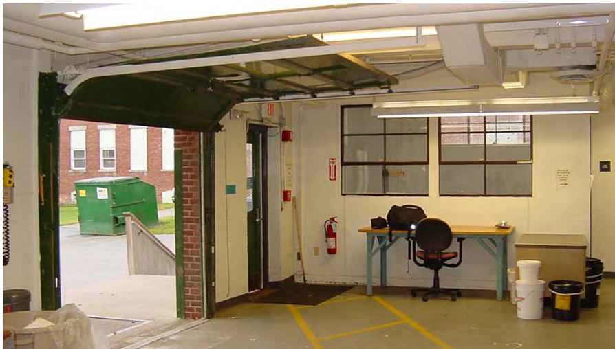
Figure 7-5. Overhead door and study room through windows
