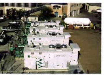
The installation of four DFC300 high temperature, highefficiency carbonate fuel cells provide the brewery virtually all of its baseload electrical power. Photo courtesy of Sierra Nevada.
