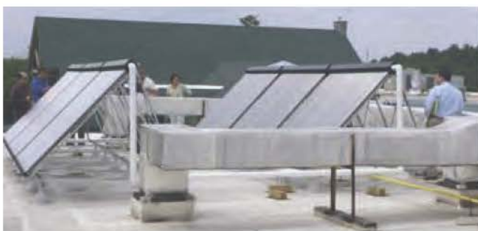
Solar thermal water system at L.L.Bean funded by a Commercial Project Grant
