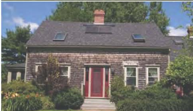
Solar Thermal System on houses in Rockport (top) and Lincolnville (bottom), both installed by ReVision Energy
