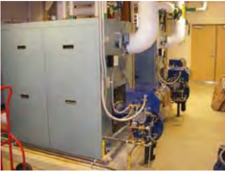
New mechanical room at the East End School, Portland, showing high-efficiency multi-stage boilers.
