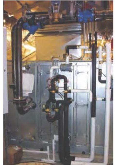
High-efficiency air handling unit at the Lincolnville Central School.
