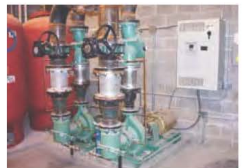
High-efficiency pump sets with variable-speed drives at the new Cony School.
