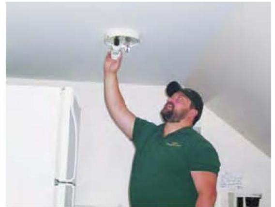
Mike Butler, Energy Auditor, Community Concepts Inc., installing a CFL bulb for a low-income customer.
