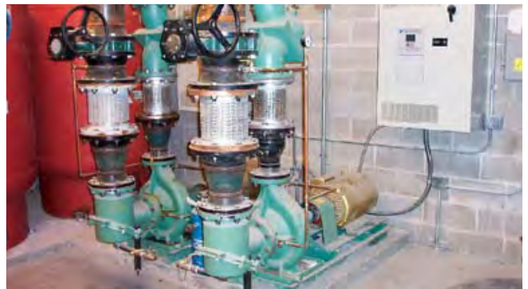
Variable frequency drive on high performance motors. Cony High School, Augusta, Maine
