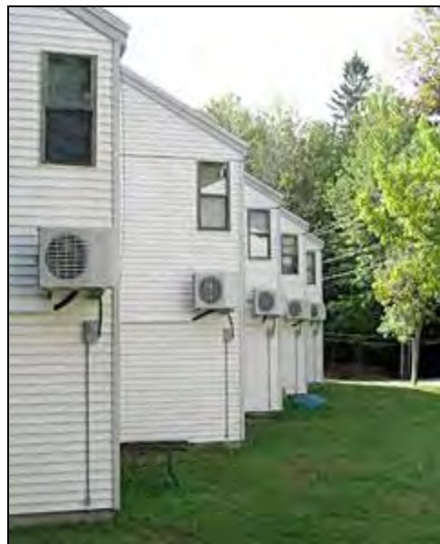
Figure 6: Multifamily heat pump installation.
