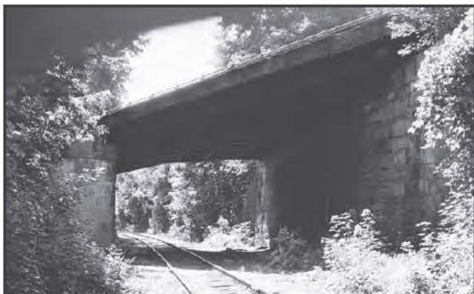
0565 Second Street Bridge, Hallowell, 1930, Replaced 2009
