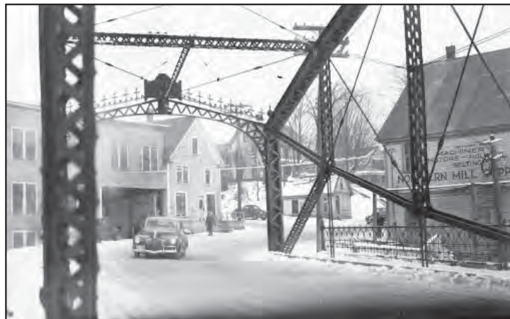
This interior view of the Old Iron Bridge in Houlton displays intricate decorative finials along the initial portal.
