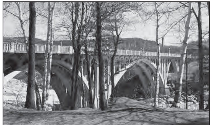
The Chisholm Park Bridge in Rumford is an open spandrel arch highway bridge. It was built from 1929 to 1930.
