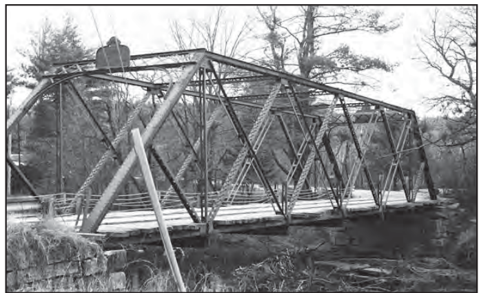
The 1921 Ryefield Bridge between Harrison and Otisfield is the only extant example of a double-intersection Warren thru truss bridge in Maine. The bridge is listed in the National Register.
