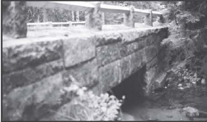
0356 UL #1 Bridge, Mt. Desert, c.1960, Replaced 2002
