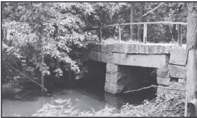
1097 Water Street Bridge, Hartland, c.1925
