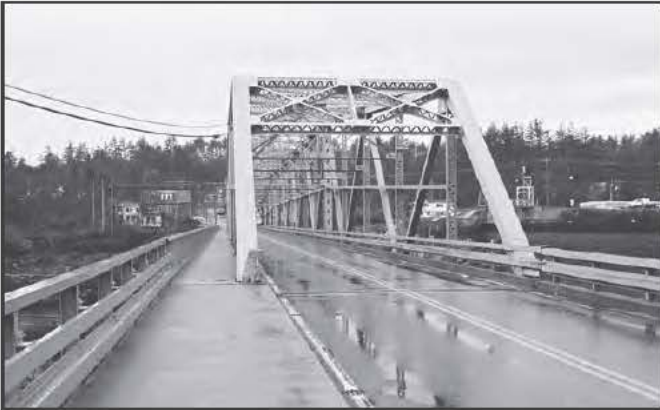
3340 West Buxton Bridge, Buxton, 1937
