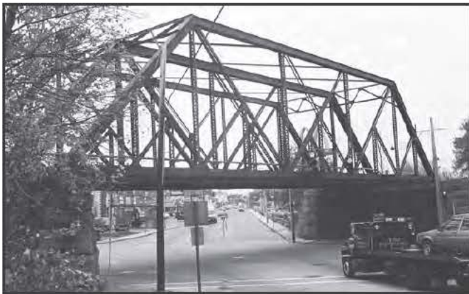
0327 St. John Street Underpass, Portland, 1890
