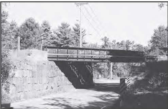
1365 Old Orchard Road Bridge, Saco, 1927
