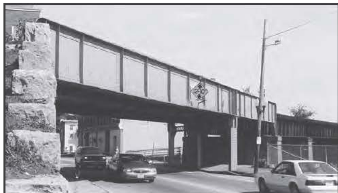
0564 Water Street Bridge Underpass Bridge, Augusta, 1914
