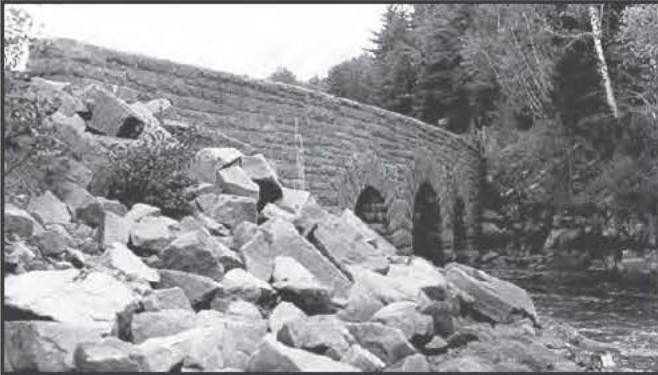
0475 Otter Creek Bridge (NPS#019P), Mt. Desert, 1938
