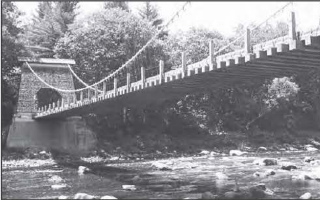
3383 Wire Bridge, New Portland, c.1866
