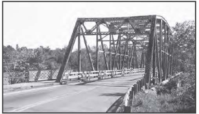
1522 Kennebec River Center Bridge, Fairfield, 1934, Replaced 2001
