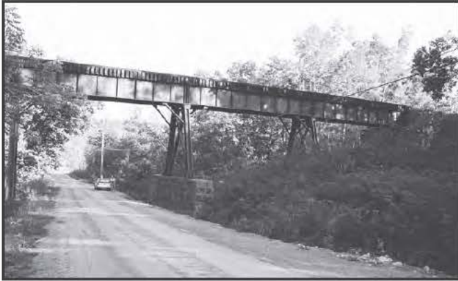
1132 Bangor & Aroostook Railroad Bridge #14.58, Frankfort, 1905
