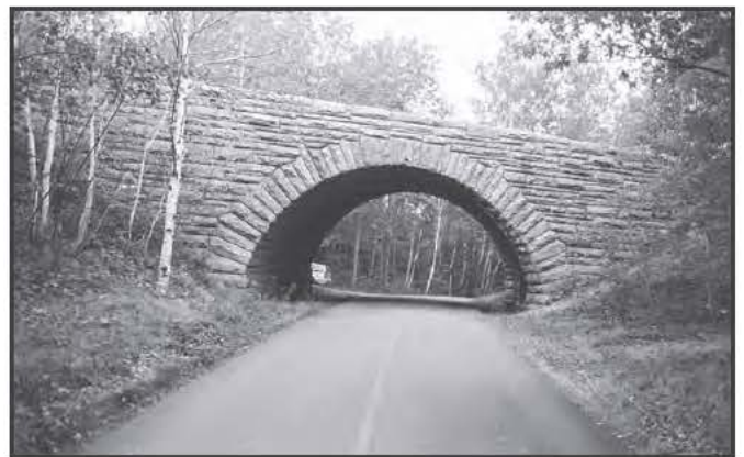
0472 Overpass Bridge (West Street-NPS#010P), Bar Harbor, 1953
