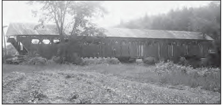
The 1876 Porter-Parsonsfield Bridge spans the Ossipee River and was built jointly by the towns of Porter and Parsonfields. Today, it is only open to pedestrians.
