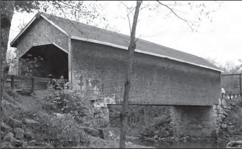
The 1876 Robyville Bridge in Corinth spans 73 feet across the Kenduskeag Stream and is the only covered bridge in the state completely covered in shingles. The Long truss bridge is a Maine Historic Civil Engineering Landmark.
