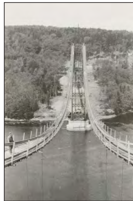
In July 1931, construction crews began stringing the cables for the Waldo-Hancock Bridge.
