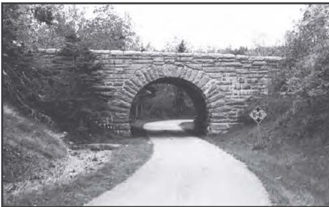
0470 Overpass Bridge (NPS#1700-002P), Bar Harbor, 1938
