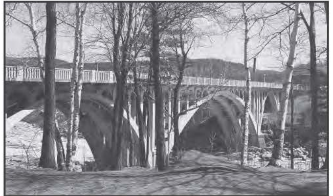
2990 Chisholm Park Bridge, Rumford, 1929
