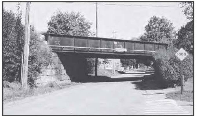
1355 James Street Bridge, Saco, 1928
