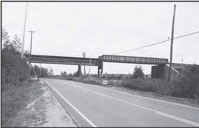
5420 Bangor & Aroostook Railroad Bridge #29.64, Hermon, 1905
