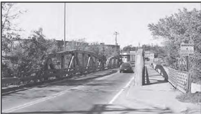
1523 Kennebec River West Bridge, Fairfield, 1934, Replaced 2001
