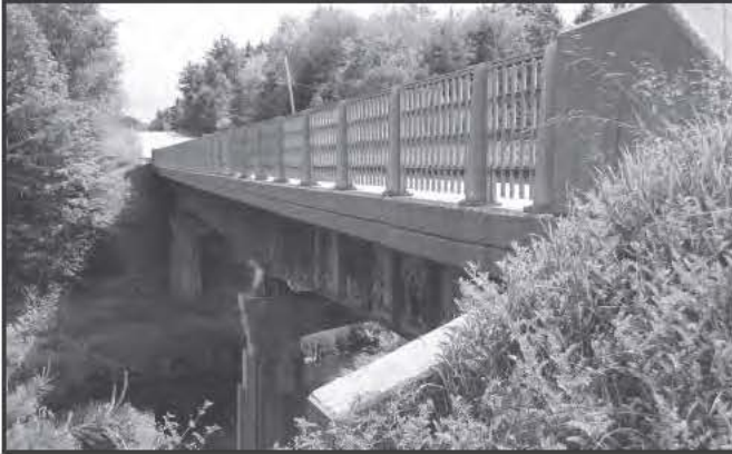
3657 Seven Mile Brook Bridge, Vassalboro, 1940
