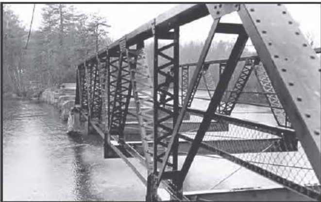
0266 Gambo Falls Bridge, Windham, 1912
