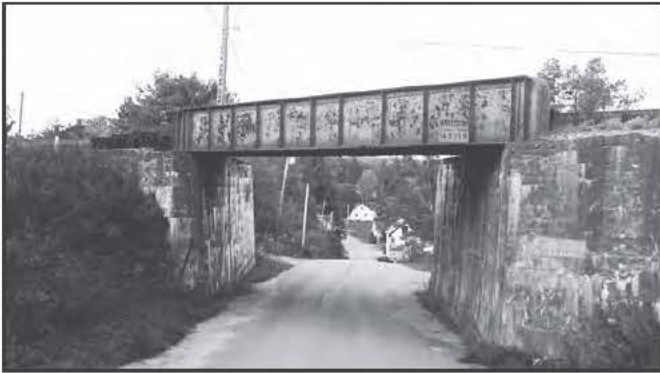
5388 Bangor & Aroostook Railroad Bridge #07.51, Stockton Springs, 1905
