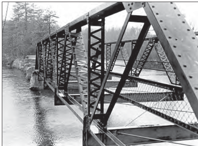
The 1912 Gambo Falls Bridge in Windham is an example of a rivet-connected Warren pony truss bridge.
