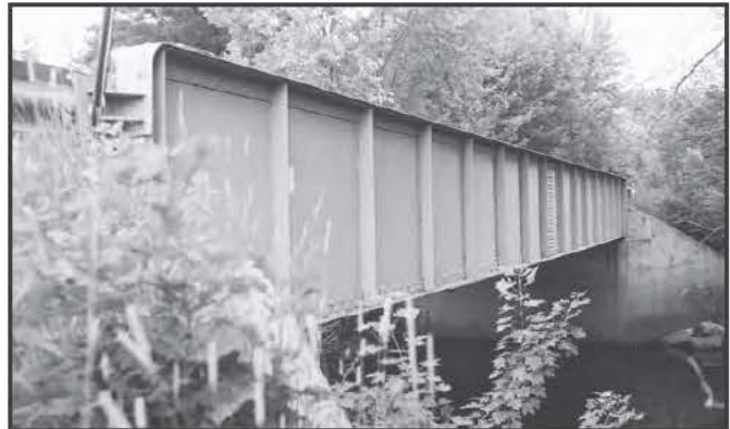
2151 Charles River Bridge, Fryeburg, 1930, Replaced 2011
