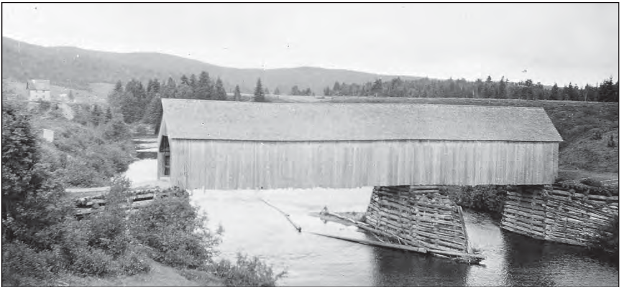
The Little Black River Bridge, shown here in 1924, in Allagash Plantation was a wooden truss bridge supported by a wood stringer span and timber crib piers and abutments. It was replaced in 1956.
