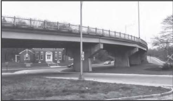
6016 Danforth Street Viaduct Bridge, Portland, 1954, Removed 2004
