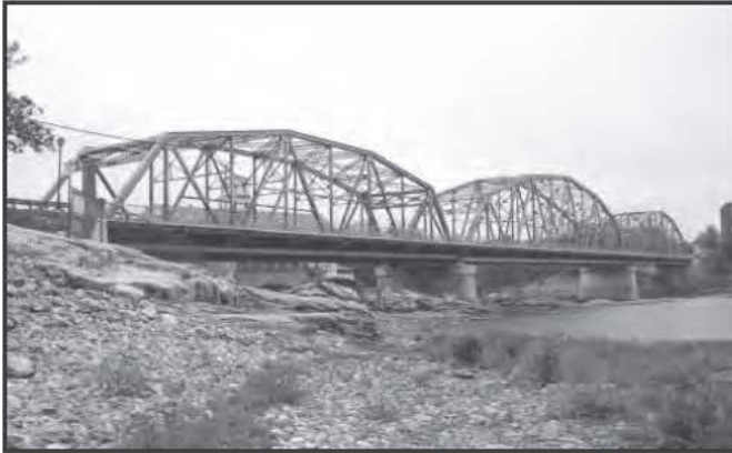
2016 Frank J. Wood Bridge, Brunswick, 1932
