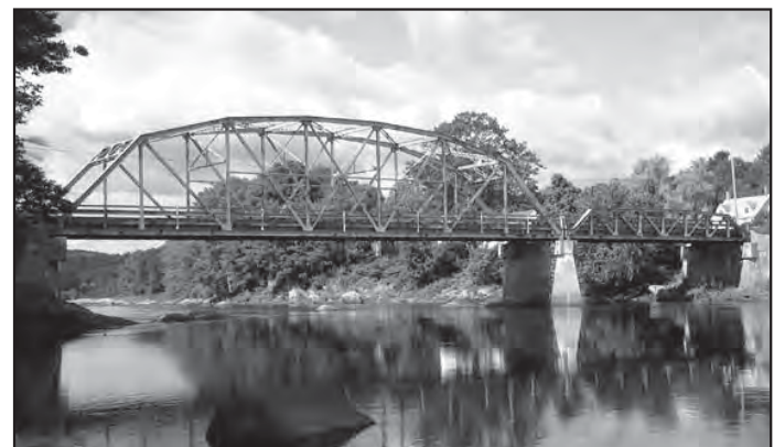
The 1936 North Turner West Bridge in Turner, replaced in 2008, was an example of a Pratt highway thru truss.
