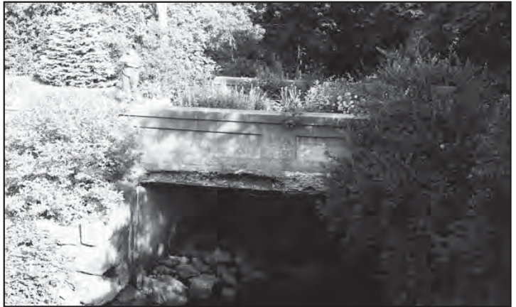
The 1909 Old Buffam Bridge in Wells is a slab bridge located on the old alignment of the Boston Post Road.
