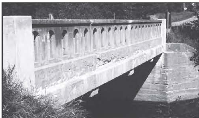
5021 Kingman Road Bridge, Macwahoc Plantation, 1919
