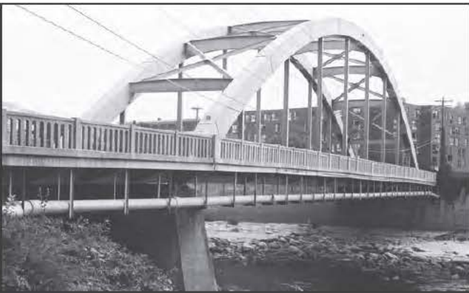
2585 Morse Bridge, Rumford, 1935
