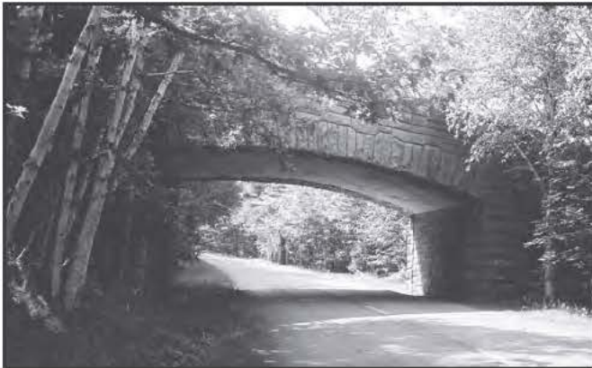
5380 Route 3 Overpass Bridge (NPS#0060), Bar Harbor, 1940
