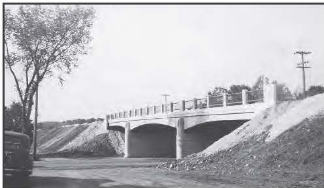
5230 Main Street Bridge, Yarmouth, 1948
