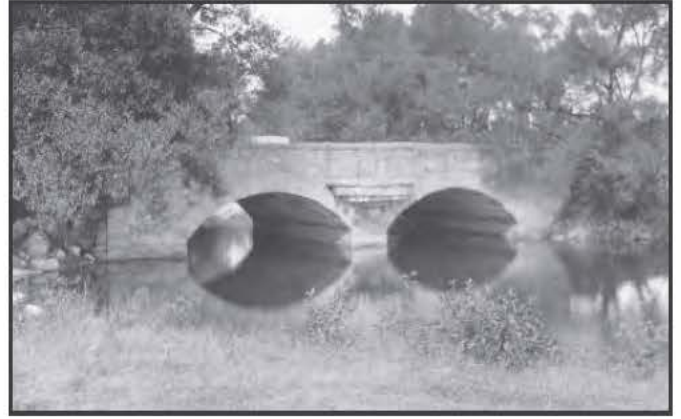
0490 Vaughan Memorial Bridge, Hallowell, 1905
