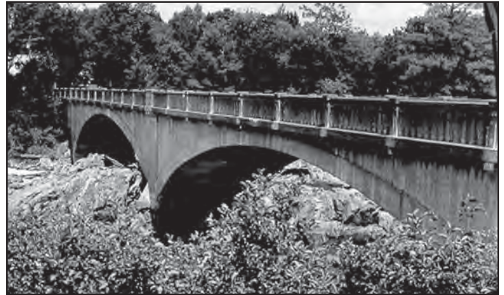
The Maine Bridge Division designed the 1923 Carrabassett Bridge in New Portland. The bridge is one of the earliest examples of a reinforced concrete bridge at this length.
