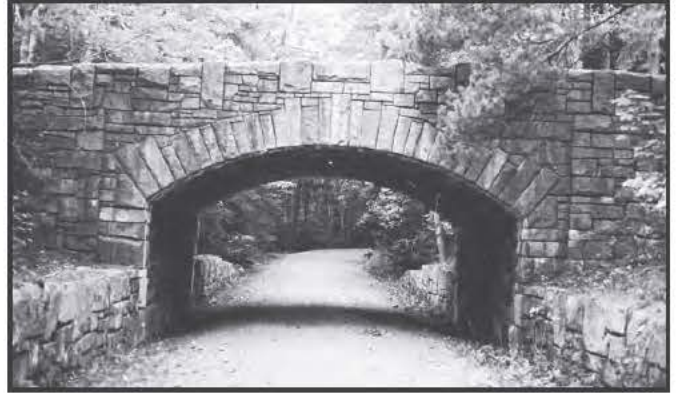
0459 Overpass Bridge, Mt. Desert, 1932
