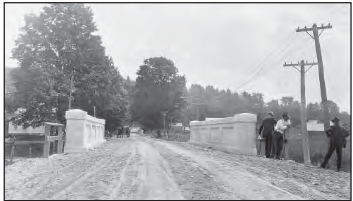
Bingham's Tom Collins Bridge, seen here in 1921, is a standard reinforced concrete thru girder type that the Maine Bridge Division used for a brief period in the early 1900s.
