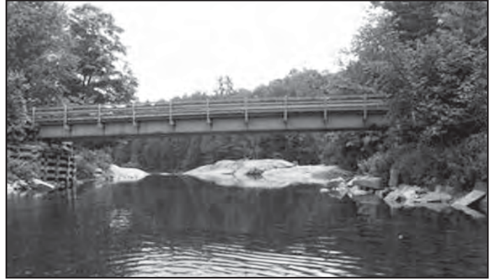
Earley's Bridge, built in 1937 in Willimantic, is a steel stringer bridge supported by a timber crib abutment.
