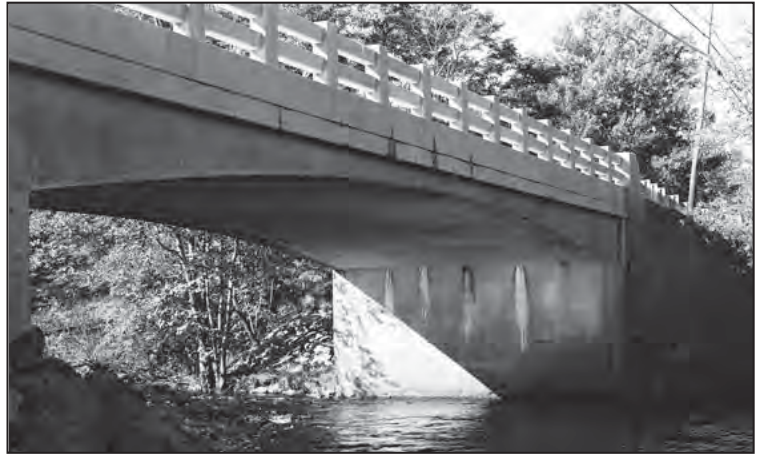
The 1935 Partridge Bridge in Whitefield illustrates the intrinsic arch profile and handsome lines that characterize the high-rise rigid frame bridge type.
