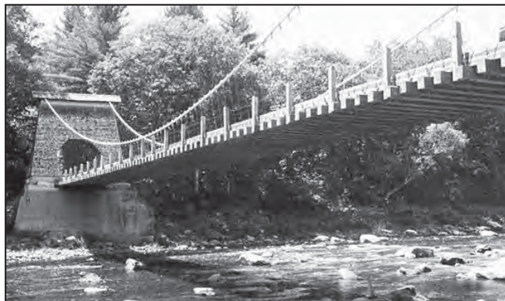
Located in New Portland, the Wire Bridge was built over the Carrabassett River from 1864 to 1866. The bridge is listed in the National Register and is a Maine Historic Civil Engineering Landmark.
