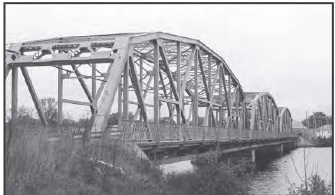
3040 Piscataquis Bridge, Howland, 1929, Replaced 2010
