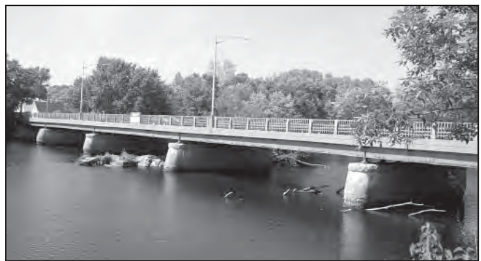
The five-span, 344-foot-long steel stringer Somesville Bridge, built in 1937 in Saco, was an early application of continuous deck design by the state bridge division.
