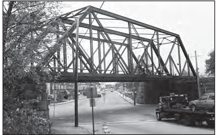
The Boston Bridge Works built the 1890 St. John Street Underpass in Portland to carry the Maine Central Railroad. The bridge is an example of a rivet-connected Baltimore thru truss.
