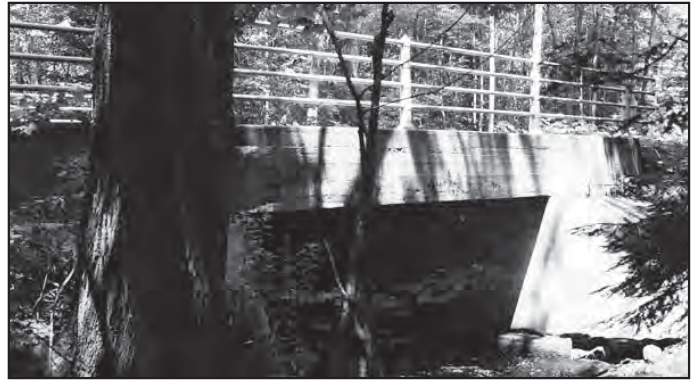
The 1920 Jellison Bridge in Sanford is a good complete example of the jack arch deck design.
