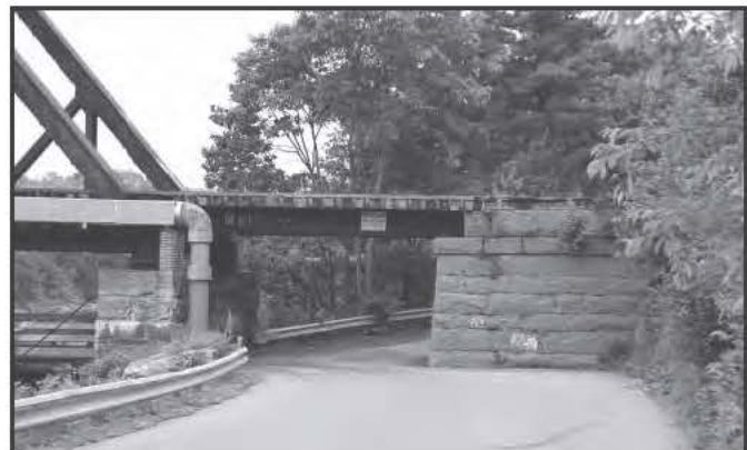
0999 Mill Road Overpass Bridge, Topsham, 1909
