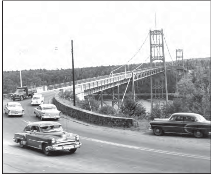
In 1956, vehicles approach and exit the 1931 Waldo-Hancock Bridge in Prospect.
