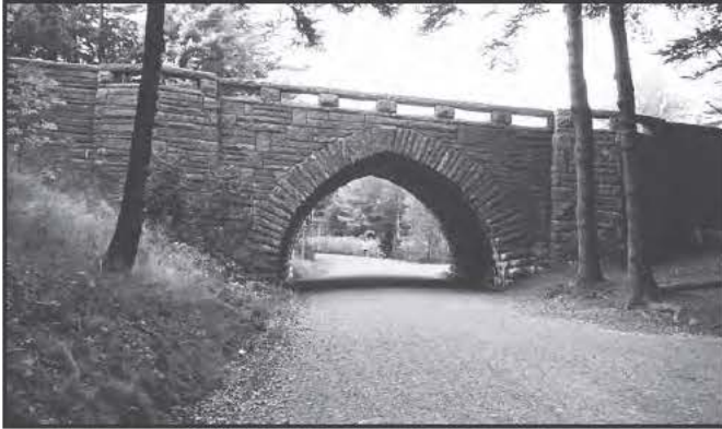
0458 Eagle Lake Road Bridge, Bar Harbor, 1928
