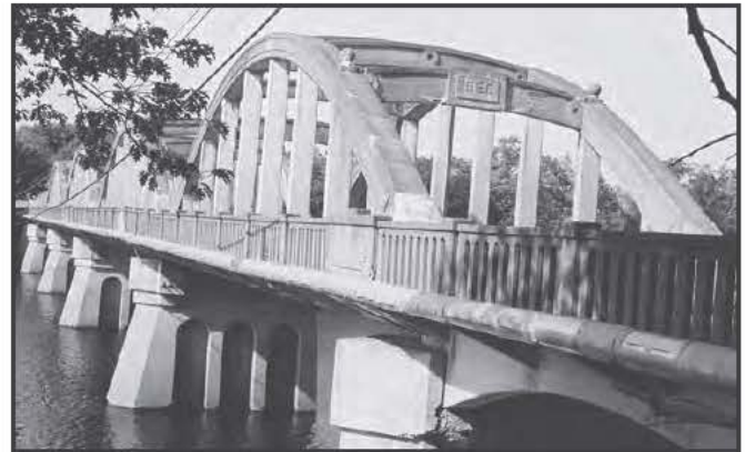
2187 Covered Bridge, Norridgewock, 1928, Replaced 2011
