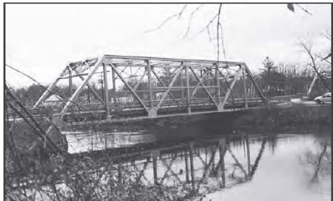
1525 Canal Bridge, Hollis, 1937, Replaced 2015
