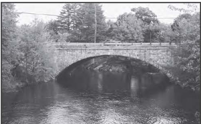
2257 East Rochester Bridge, Lebanon, 1946
