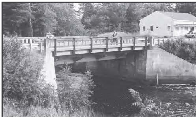
2674 Pleasant River Bridge, Columbia Falls, 1920
