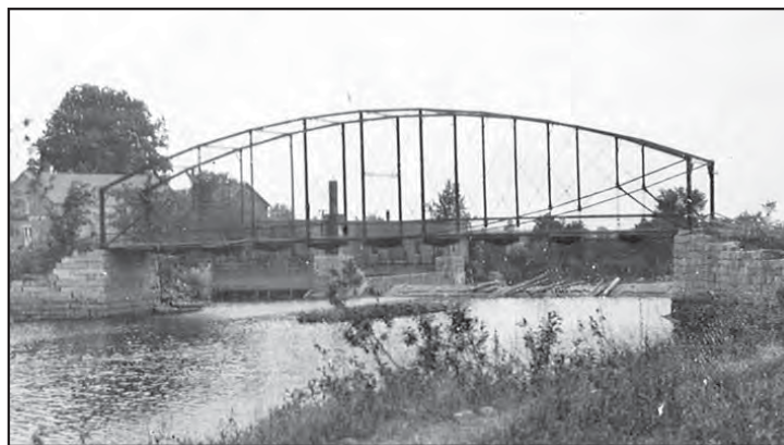
The East Dover Bridge in Dover-Foxcroft exemplified the Lenticular truss, a popular iron bridge type in the 1870s through 1890s.
