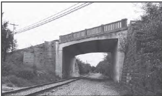
3172 Railroad Crossing Bridge, Freeport, 1936
