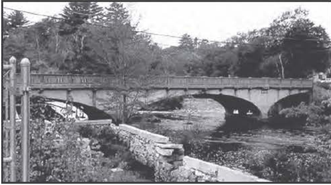
2432 Kezar Falls Bridge, Parsonsfield, 1924, Replaced 2000
