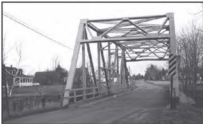
2565 Mill Pond Bridge, Salem Township, 1929, Replaced 2004
