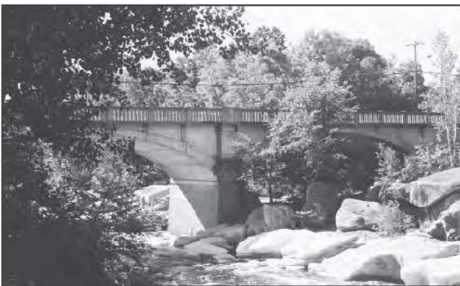
5063 Lower Village Bridge, Phillips, 1927
