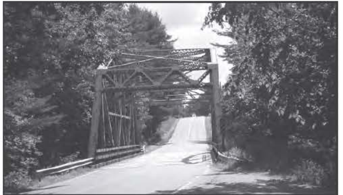
3214 North Turner East Bridge, Leeds, 1936, Replaced 2008
