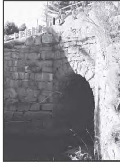
2560 Mill Creek Bridge, Falmouth, 1894
