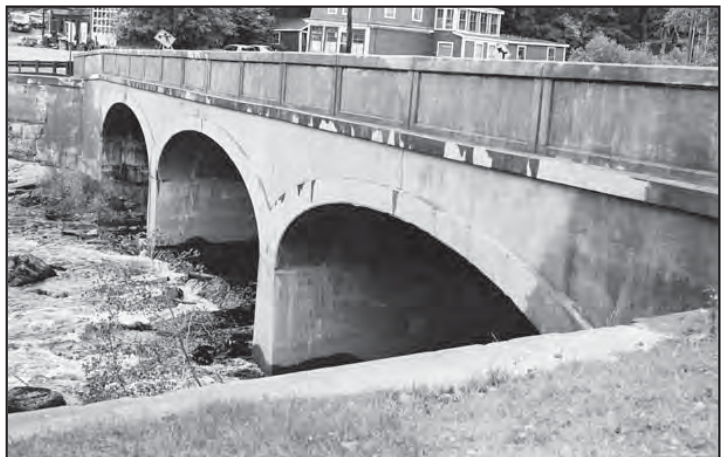
The 1902 Pope Memorial Bridge in East Machias is Maine's oldest reinforced concrete deck arch bridge.
