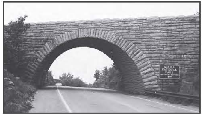
0471 Mountain Road Underpass Bridge (NPS#020P), Bar Harbor, 1951
