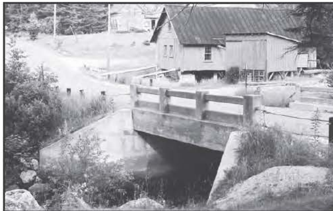
3590 Andrews Bridge, Woodstock, 1938
