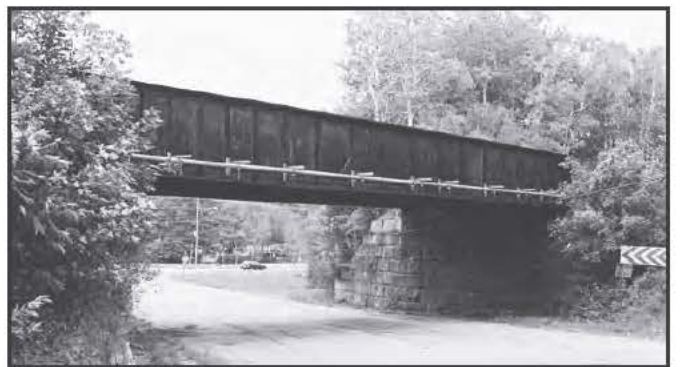
5337 Boston & Maine Railroad Underpass Bridge, Wells, 1920
