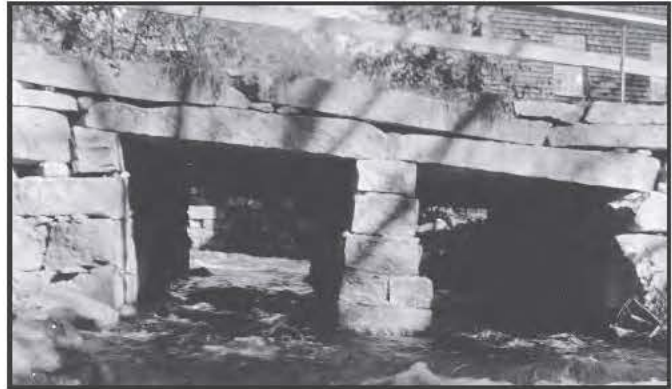
0747 Watson's Bridge, Waterford, 1890
