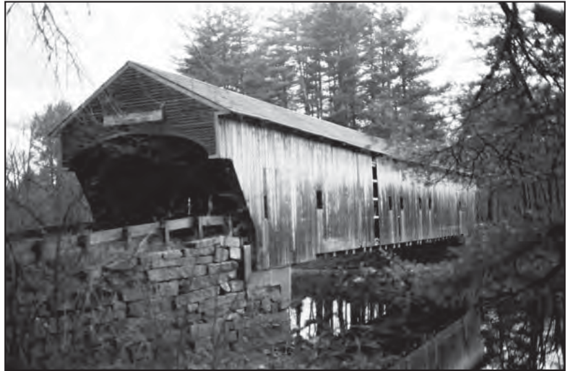
The 1857 Hemlock Bridge in East Fryeburg spans the Old Course of the Saco River. The 109-foot long Paddleford truss bridge carries local traffic and is the oldest extant covered bridge in Maine.
