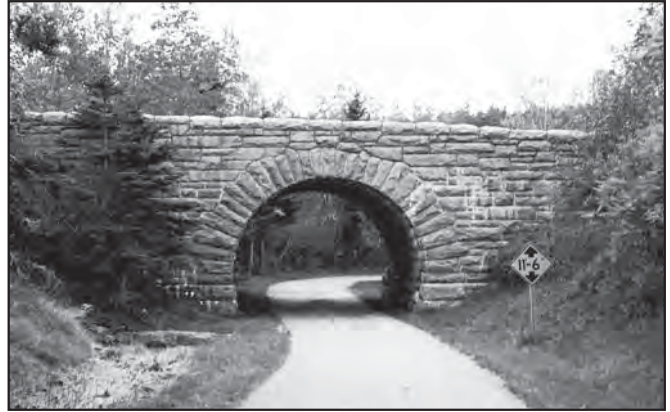
This signature, stone-faced, reinforced concrete arch bridge is in Acadia National Park. John D. Rockefeller, Jr. had the bridge built as part of a system of grade-separated carriage and motor roads.
