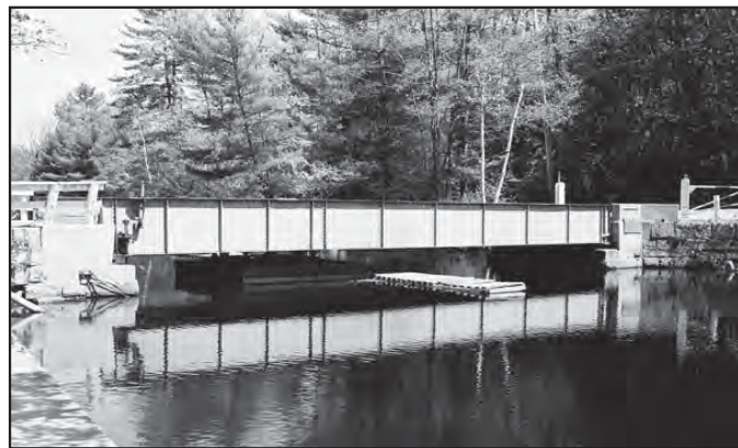
The 1901 Songo Lock Draw Bridge is sixty-feet long moveable bridge. It has a hand-operated center-bearing bobtail swing span.
