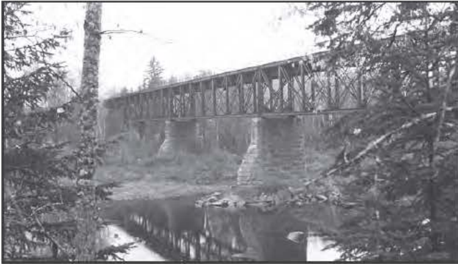
0159 Bangor & Aroostook Railroad Bridge #A44.74, Ashland, 1902
