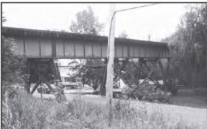
1130 Bangor & Aroostook/Monroe Road Railroad Bridge #1603, Frankfort, 1905
