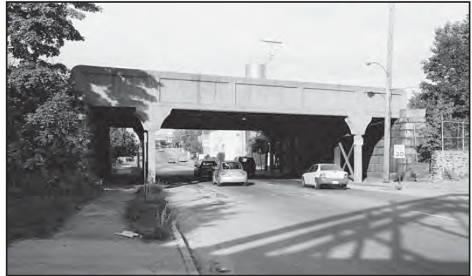
The 1890 Park Avenue Underpass in Portland is an early surviving example of a girder-floorbeam bridge with concrete encasement to protect the beams.
