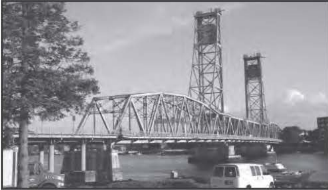
2546 Memorial Bridge, Kittery, 1921, Replaced 2013
