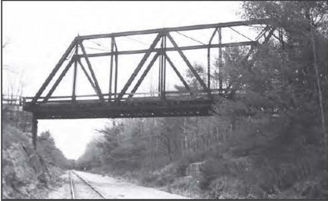
0210 Overpass Bridge, Yarmouth, 1888, Replaced 1999
