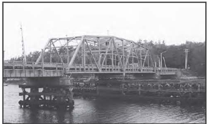
2789 Southport Bridge, Southport, 1939
