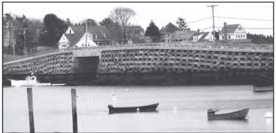
Edwards designed the one-of-a-kind Bailey Island Bridge, his most enduring and iconic structure.
