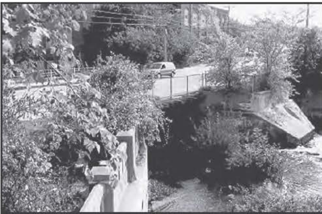
1359 Washington Street Bridge, Sanford, 1911
