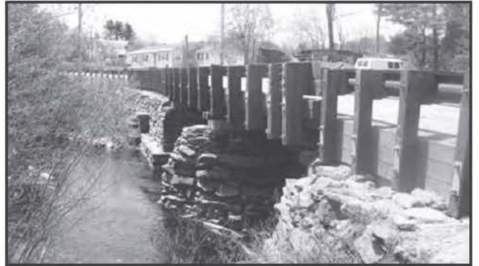
5258 Grist Mill Bridge, Lebanon, c.1790
