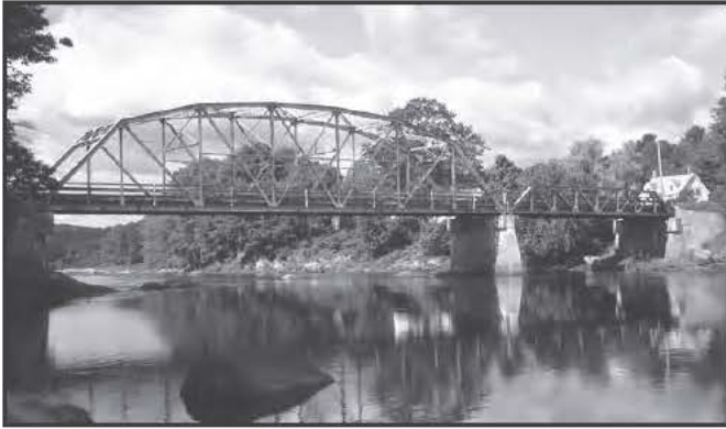
1474 North Turner West Bridge, Turner, 1936, Replaced 2008
