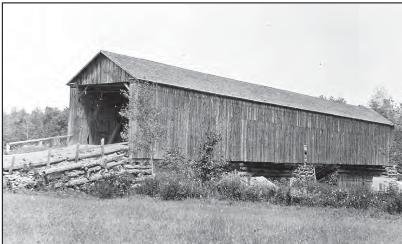
Located in Littleton, the c.1903 Watson Bridge spans the Meduxnekeag Stream and is the only extant Howe truss covered bridge in Maine. This bridge is a Maine Historic Civil Engineering Landmark.
