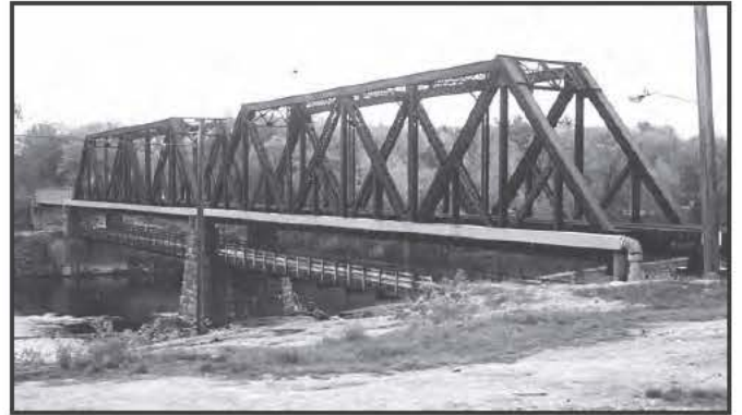
0323 Free/Black Bridge, Brunswick, 1909, Lower Deck Removed 2014
