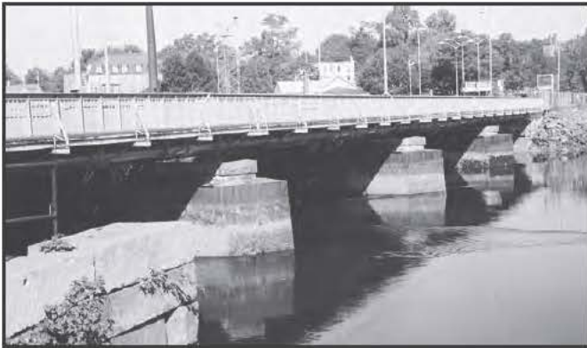
1357 Navy Yard Entrance Bridge, Kittery, 1919
