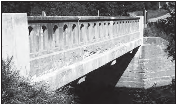
The 1919 Kingman Road Bridge in Mawahoc Plantation is among the earliest, state-built T-beam bridges in Maine.
