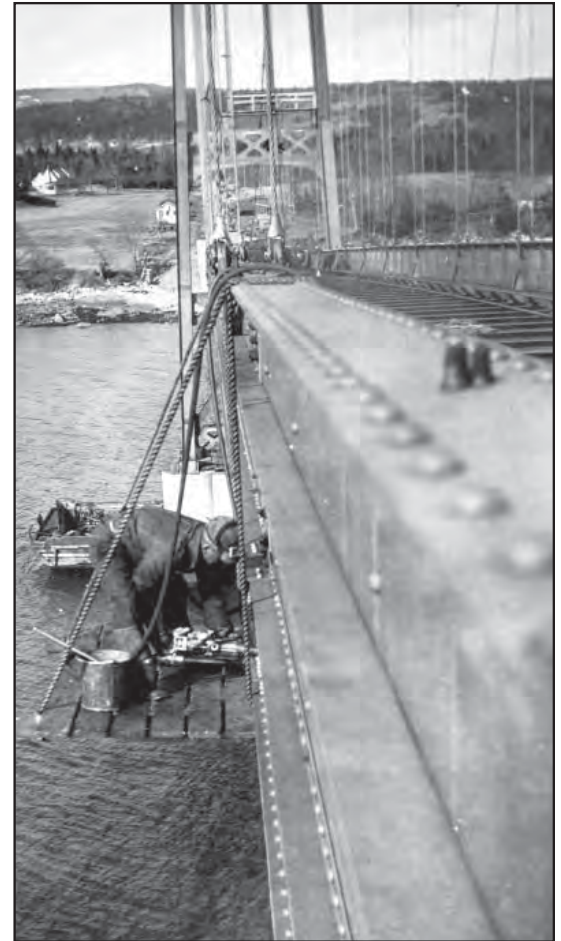
A riveter works on the Deer Isle-Sedgwick suspension bridge in 1939.
