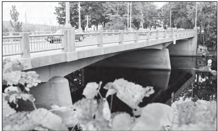
The Mechanic Falls Bridge, built in 1949 in Mechanic Falls, is one of Maine's earliest multiple-span, high-rise rigid frame bridges.
