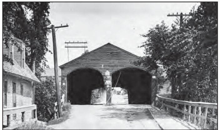
The Big Stillwater Bridge was an example of a double-barrel covered bridge which utilized the Town truss system. This bridge was located near Orono and was replaced in 1951.
