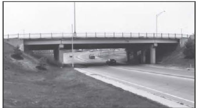
6015 B Road Overpass Bridge, Portland, 1954, Removed 2004
