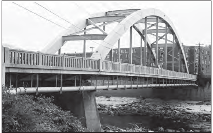
The 1935 Morse Bridge in Rumford is the only example in Maine of a steel tied thru arch. It also bears a concrete arcade railing.
