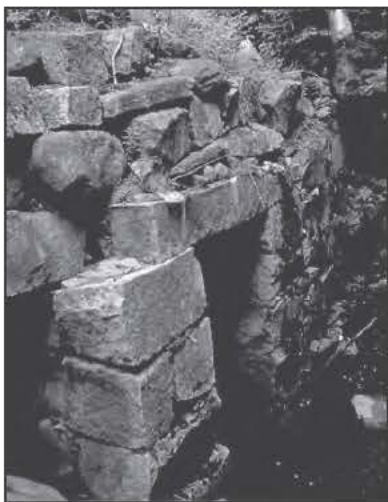
0403 McLeary Brook Bridge, Strong, c.1879
