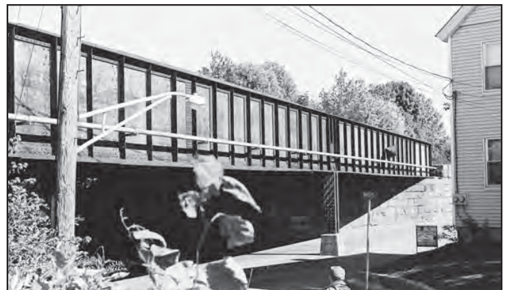
Built from 1927 to 1928 in Saco, the Common Street Bridge illustrates the ubiquitous girder-floorbeam technology used by railroads across Maine and the nation.
