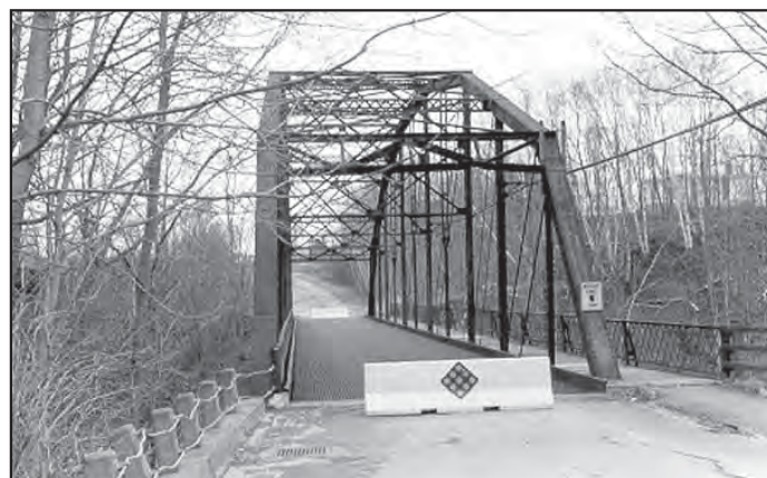
The 1916 New Sharon Bridge in New Sharon was the last pin-connected bridge in Maine. The former National Register-listed bridge was a Pennsylvania thru truss.
