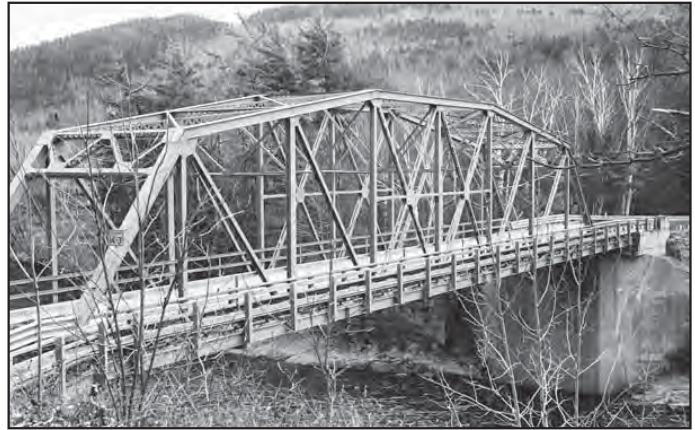
Gilead's Androscoggin River Bridge, built in 1921, is an exceptional example of a Parker camelback truss bridge.
