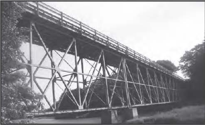
3016 Back River Bridge, Arrowsic, 1933, Replaced 2007
