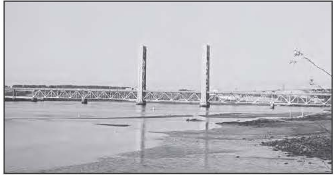
3641 Sarah Mildred Long Bridge, Kittery, 1940, Replaced 2015
