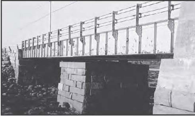
1475 Great South Bridge, Milbridge, 1936, Replaced 2010
