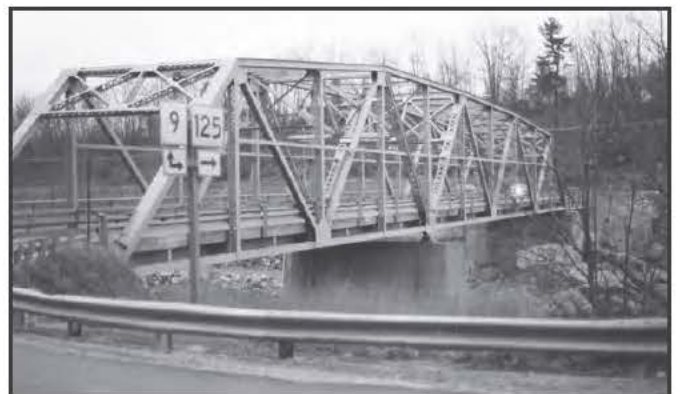
3334 Durham Bridge, Durham, 1937, Replaced 2015
