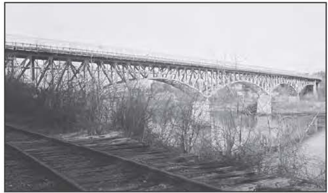
5196 Memorial Bridge, Augusta, 1949
