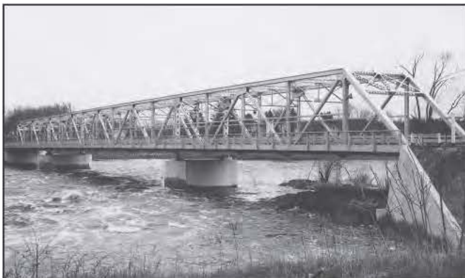
3333 Bar Mills Bridge, Hollis, 1937, Replaced 2015
