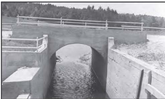
3876 Johnsons Mill Bridge, Waterboro, 1920*
