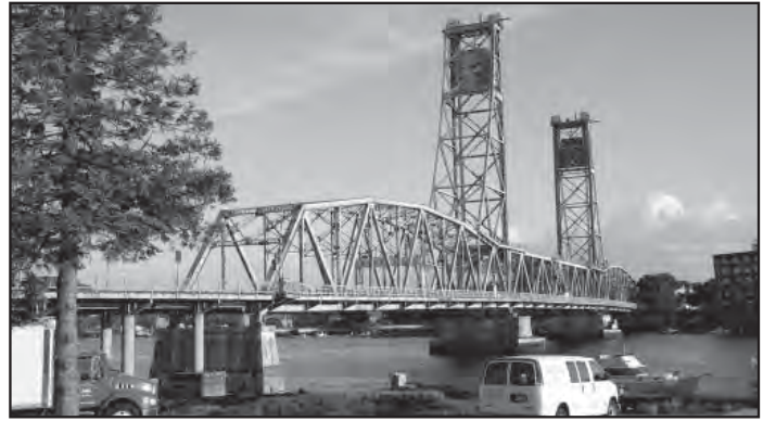
Prominent bridge engineer J. A. L. Waddell designed Memorial Bridge, a vertical lift span built from 1920 to 1921 in Kittery. The bridge was removed in 2012.
