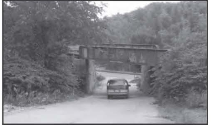
1136 Bangor & Aroostook Railroad Bridge #15.61, Frankfort, 1905
