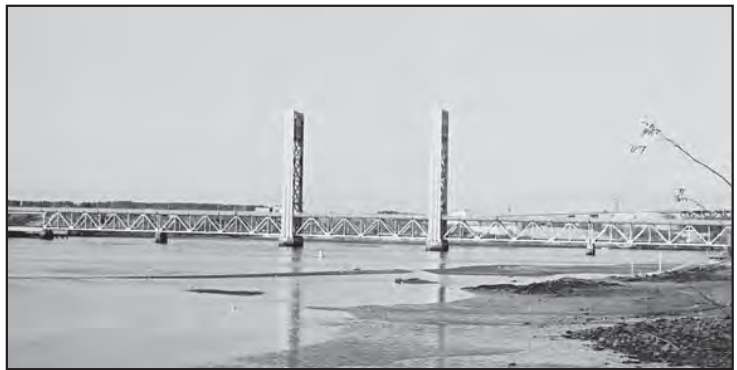
The 1940 Sarah Mildred Long Bridge in Kittery was a vertical lift bridge with electric drive motors and Art Moderne-style towers.
