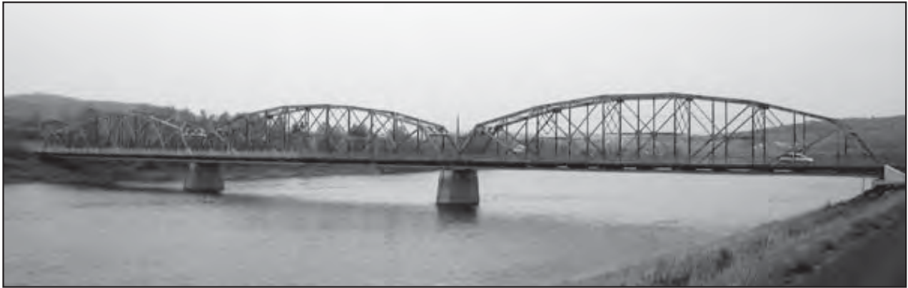
Once located in Fort Kent, the three-span 1929 International Bridge was an example of the Pennsylvania truss.
