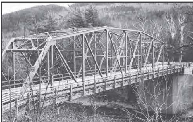
5084 Androscoggin River Bridge, Gilead, 1921
