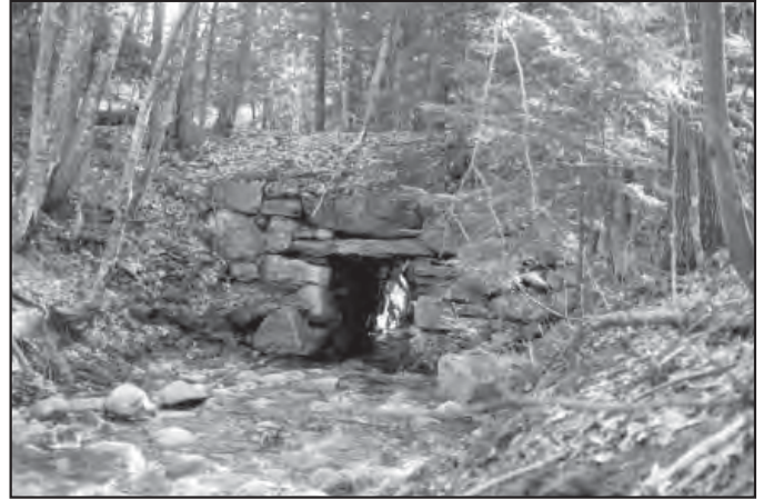
The 1797 Churchill Bridge near Buckfield is a rare stone slab bridge. Courtesy of Maine Historic Preservation Commission
