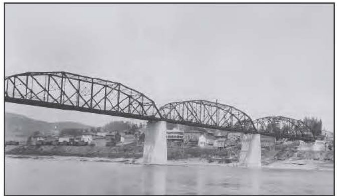
2399 International Bridge, Madawaska, 1921
