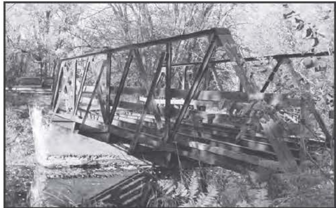
1022 Bailey Bridge, Harmony, 1915, Removed 2000
