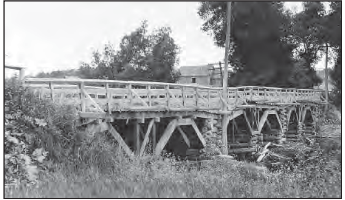
The Red Bridge in Houlton, pictured here in 1924, consisted of stacked timber piles and an uncovered wooden deck.
