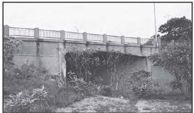
3525 Danforth Street Crossing Bridge, Portland, 1939
