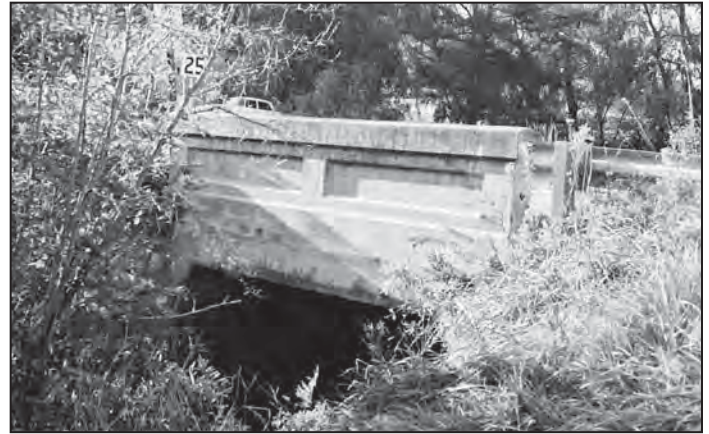
Located in Union, Young's Bridge, built in 1917, is the earliest identified example of the standard low-rise rigid frame bridge used by the Maine State Highway Commission.
