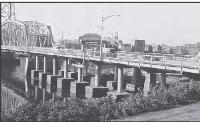
5276 Viaduct Bridge, Kittery, 1921, Replaced 2012
