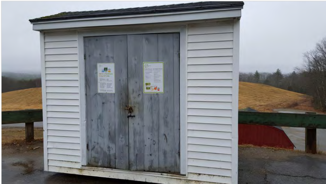
PaintCare provided signage shown on the paint shed at the Waldoboro Transfer Station.
