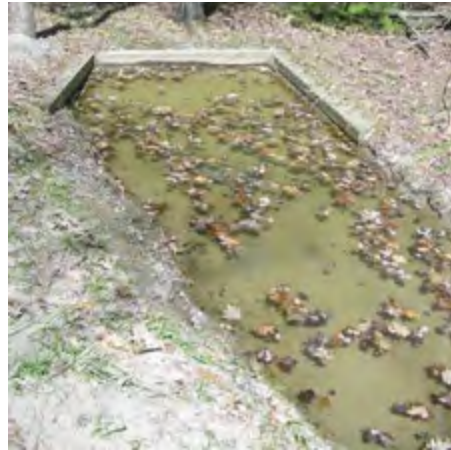
The above photo shows a typical level spreader used to evenly disperse flows to a vegetated area.
