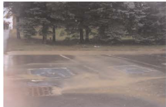
This parking area contributes sediment to the storm drain network, where it will be carried to the nearest surface water. The sediment contains many pollutants that are deposited through air pollution or directly by cars, as these have a tendency to stick to the sediment particles. Sediments fill in waterbodies, providing a substrate for aquatic weed growth, and can have an adverse effect on fish and other organisms.
