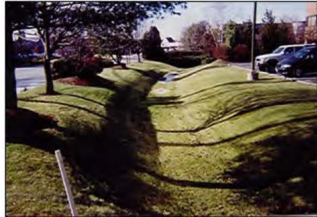
This dry swale is located in New Hampshire. It blends well with the landscaping and is low maintenance yet effective. It does have an overflow to the storm drain system that can be accessed once the water reaches more than halfway up the side slopes.
