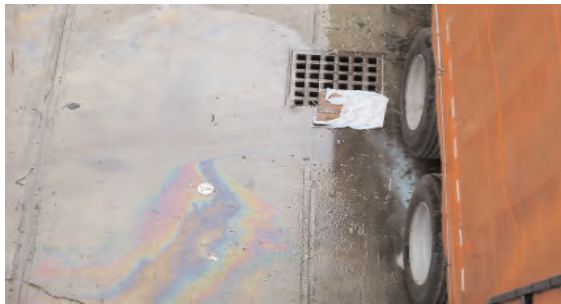
This oil sheen, left by parked vehicles, makes its way towards this catch basin and storm drain network. Without proper treatment, the oil will enter the nearest surface water, where it will degrade fisheries habitats.
