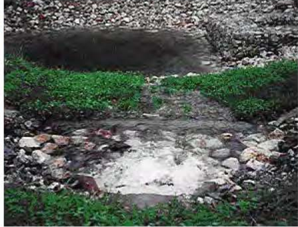
This pretreatment basin or sediment forebay has simple construction using a gabion (rock filled wire basket) berm. This helps reduce the velocity of the flows and settle out some sediments before the water is treated further.
