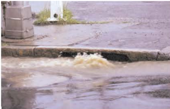
The photo above shows runoff from a developed area entering a municipal storm drain system. If not managed properly, increased runoff can flood local roads and waterways, as the capacity of drainage structures and natural channels are taxed.
