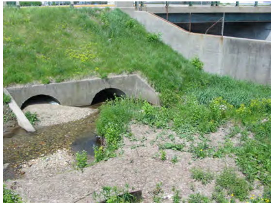
These culverts are preceded by a small detention area, which has filled in with sediment due to lack of maintenance. As a result, sediment is transported from this area further downstream during storms events. Improvements to increase the detention area could easily be made, however, periodic maintenance is crucial to the performance of the BMP.
