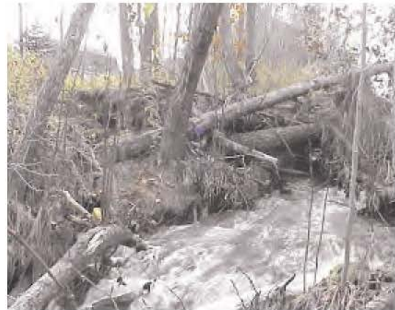
Increased streamflow volumes and velocities associated with urban impacts have resulted in significant erosion of streambanks, as shown here in Bangor, Maine.
