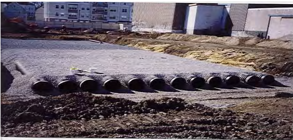
Subsurface detention and infiltration galleries, where feasible, like this one have become popular in recent years due to their space saving location under the parking lot. With visible and adequate pretreatment and frequent maintenance, they can work well and will help recharge groundwater. However, many designs today do not have pretreatment and are difficult to clean out, so they quickly fill with sand and fail. The pollutants they were supposed to treat then go out to water bodies or into the municipal system where taxpayers foot the bill for maintenance.
