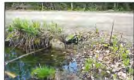
Crushed culvert identified in survey
