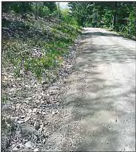
Scouring of ditch. Long run with no cross culverts or turnouts.
