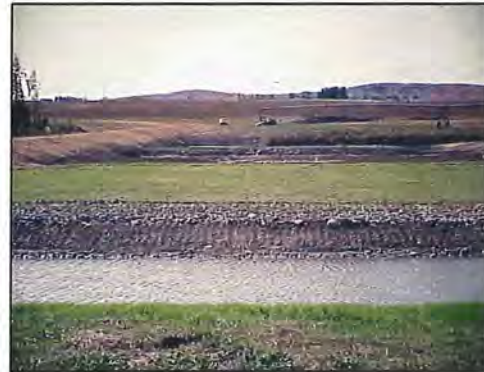
Nutrient & sediment control structure under construction.
