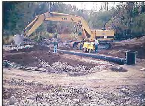
Construction of pond and outfall components of nutrient and sediment control system
