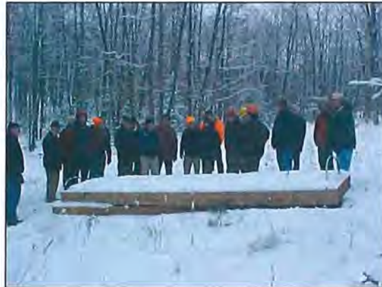
Swamp crane mats were installed to minimize soil disturbance by skidders in sensitive/wet areas.
