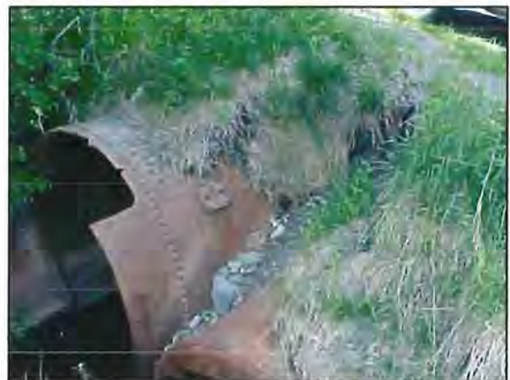
Soil erosion around town road culvert
