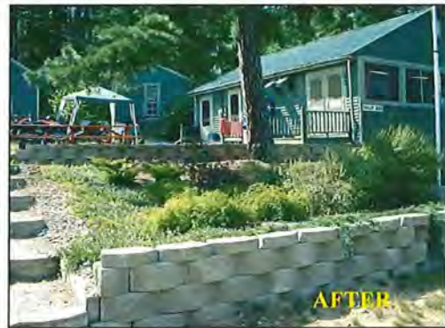
Kiwanis Beach – 38 volunteers from local businesses, garden clubs, Kiwanis and the WLA chipped in to plant shrubs, build infiltration steps, repair failed retaining walls, and install a drywell.
