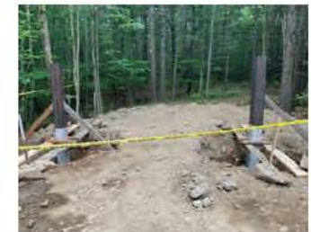
Entrance roughed in and holes for gate posts dug.
