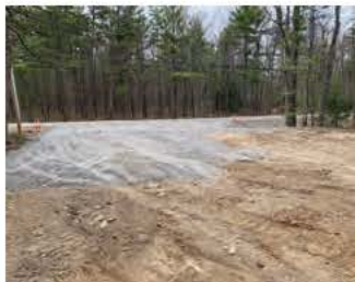
Fill for the access road was brought in and the posts set.
