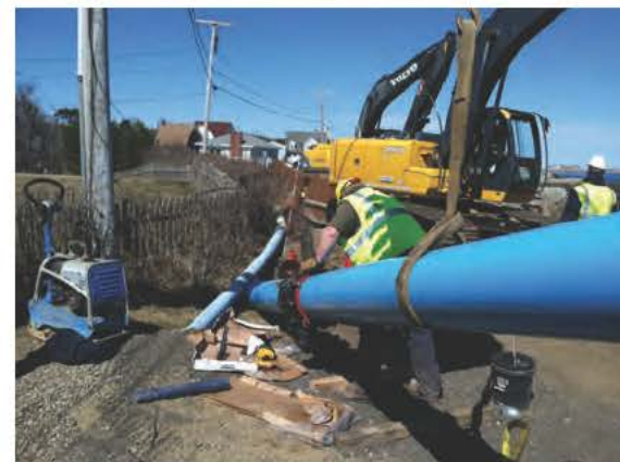
Water main replacement at Kennebunk, Kennebunkport and Wells Water District.
