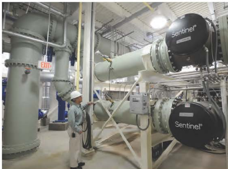
Ultraviolet (UV) disinfection system at Auburn Water District
