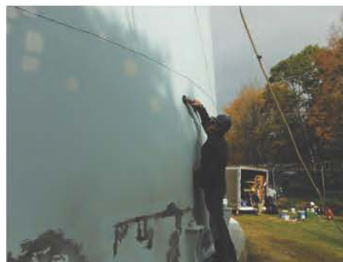
Repair on the Mount Pisgah Standpipe in preparation for painting at Boothbay Region Water District
