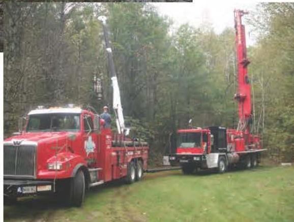
Installation of a new well at Solon Water District
