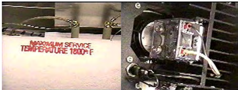
e. Furnace and connections
