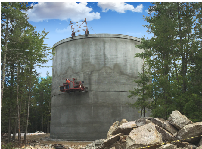
Kennebunk, Kennebunkport & Wells Water District's new 1.5 million-gallon water storage tank in Arundel was completed in 2021 with DWSRF funds. (Photo: McKenzie Parker)
