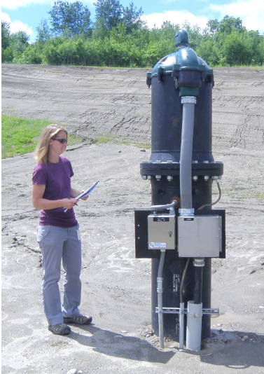
Municipal public water system inspector, Denise Douin, inspects Greater Augusta Utility District's well on a sanitary survey.
