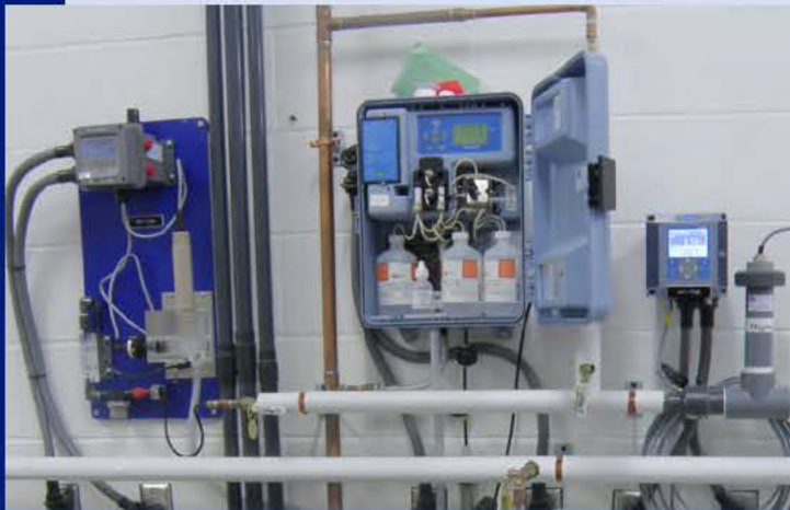
In-line analyzers continually monitor fluoride, chlorine and pH levels in the drinking water at drinking water treatment plant.
