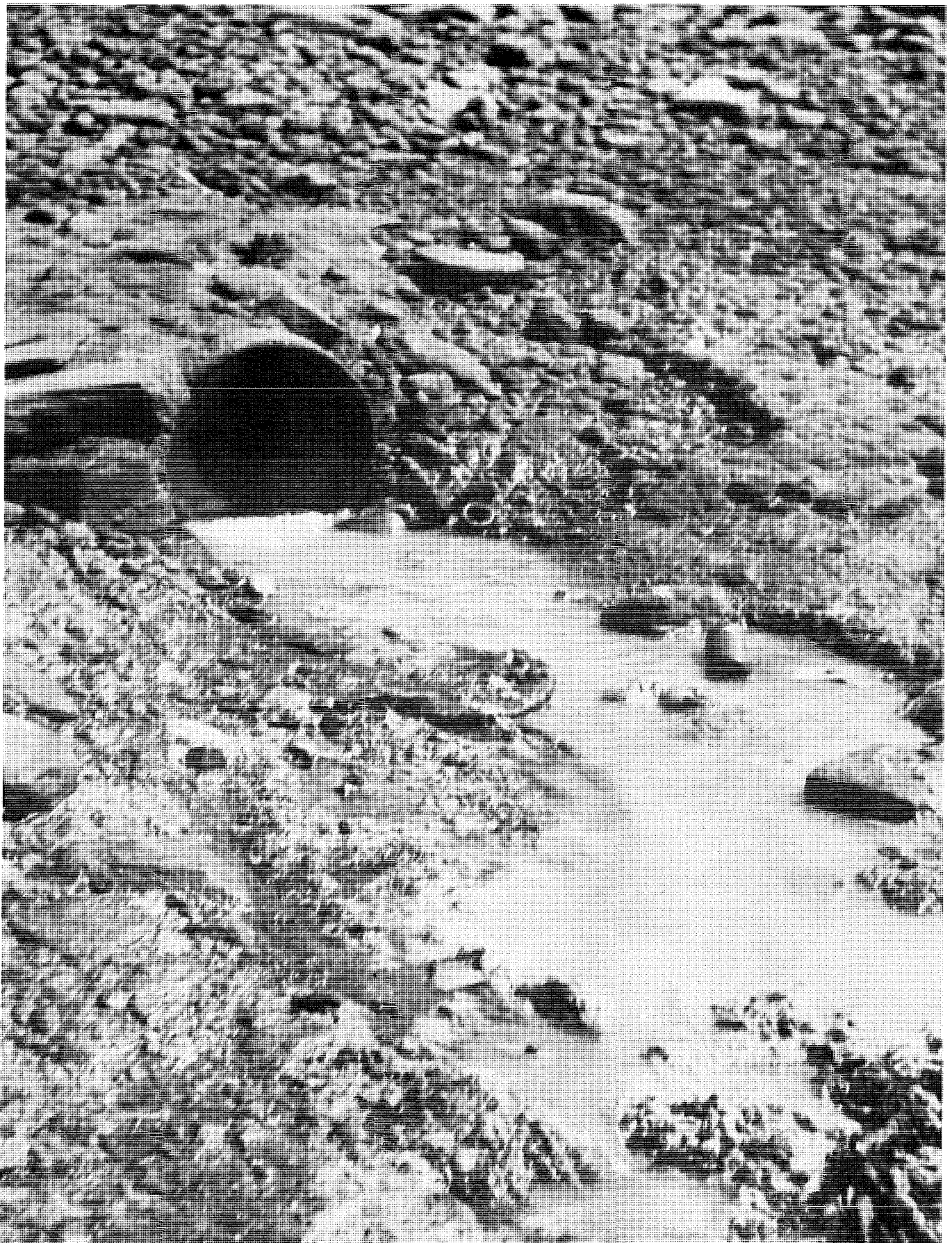
TEN INCH PUBLIC SEWER OUTFALL DISCHARGING SANITARY WASTES TO TIDEWATER AT MOUTH OF PENOBSCOT RIVER.
