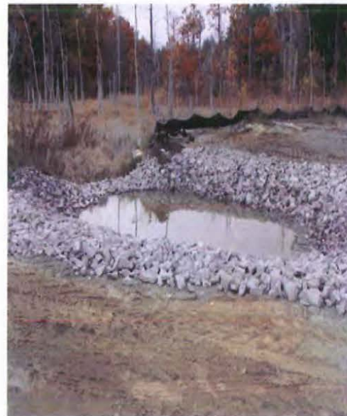
Solution: Install rock lined plunge pool to control sediment from entering the wetland.
