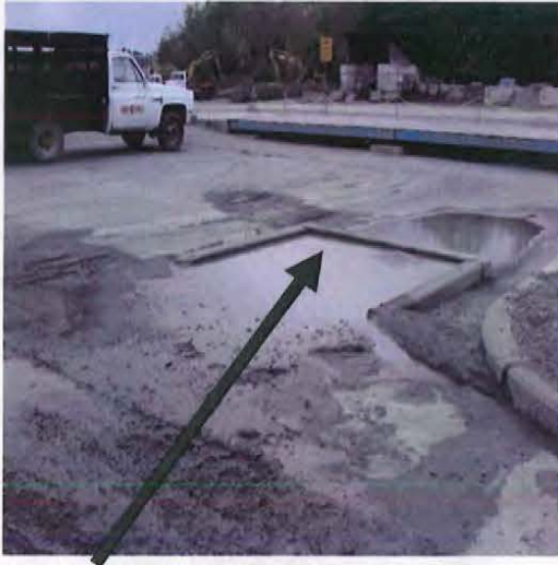
Problem: Stormwater catch basin located in maintenance area drains to the Penobscot River.
