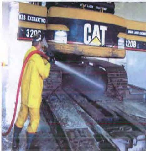
Problem: Although an activity is performed inside, the impact to stormwater can still be significant if the material is allowed to be tracked or washed out of a door.
