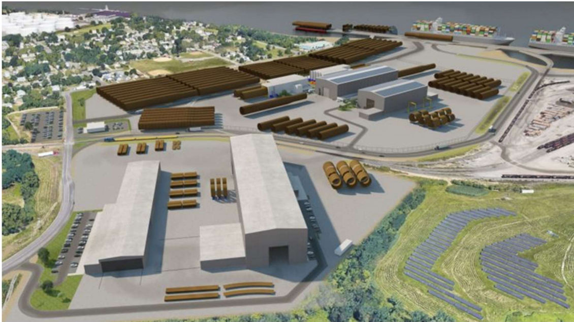
Figure 3-12. Planned monopile fabrication facility in Paulsboro, New Jersey (Source: NJEDA)
