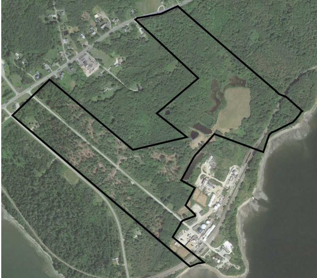
Figure 5-4: Available Area at GAC Chemical Site
