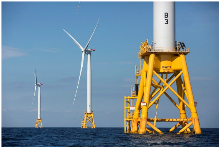
Figure 1-1: Block Island Wind Turbines with Jacket Foundations (Source: Vineyard Wind).
