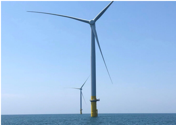
Figure 1-2: Coastal Virginia Wind Turbines with Monopile Foundations (Source: Dominion Energy)
