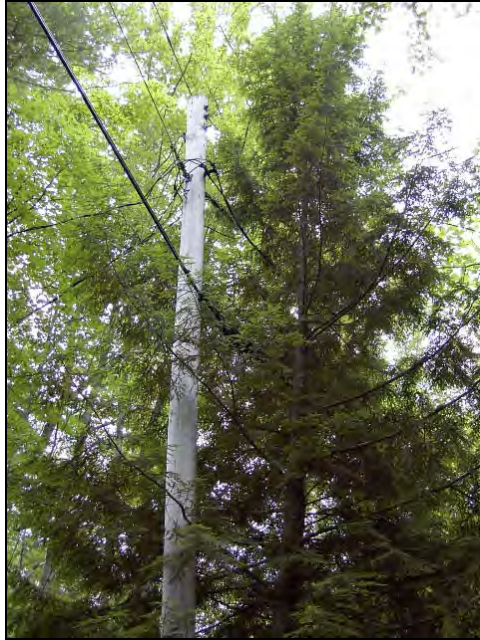
Heavy vegetation in contact with 1-phase circuit
