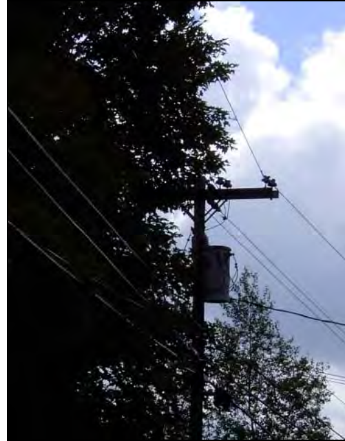
Heavy vegetation in contact with 3-phase circuit
