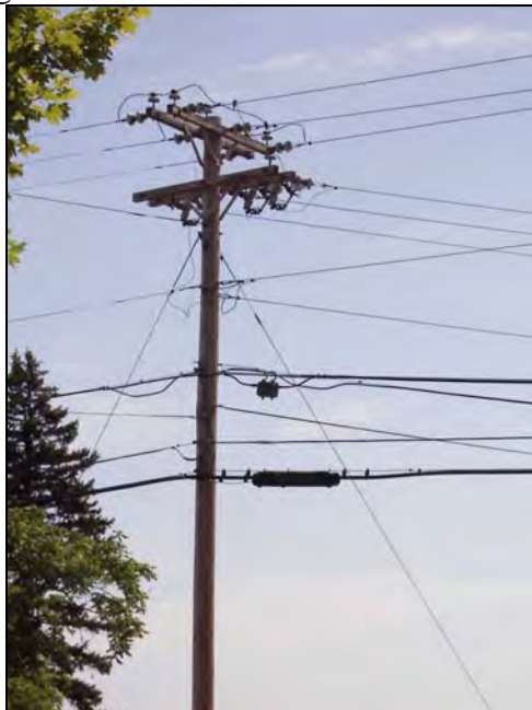
Typical 3-phase pole
