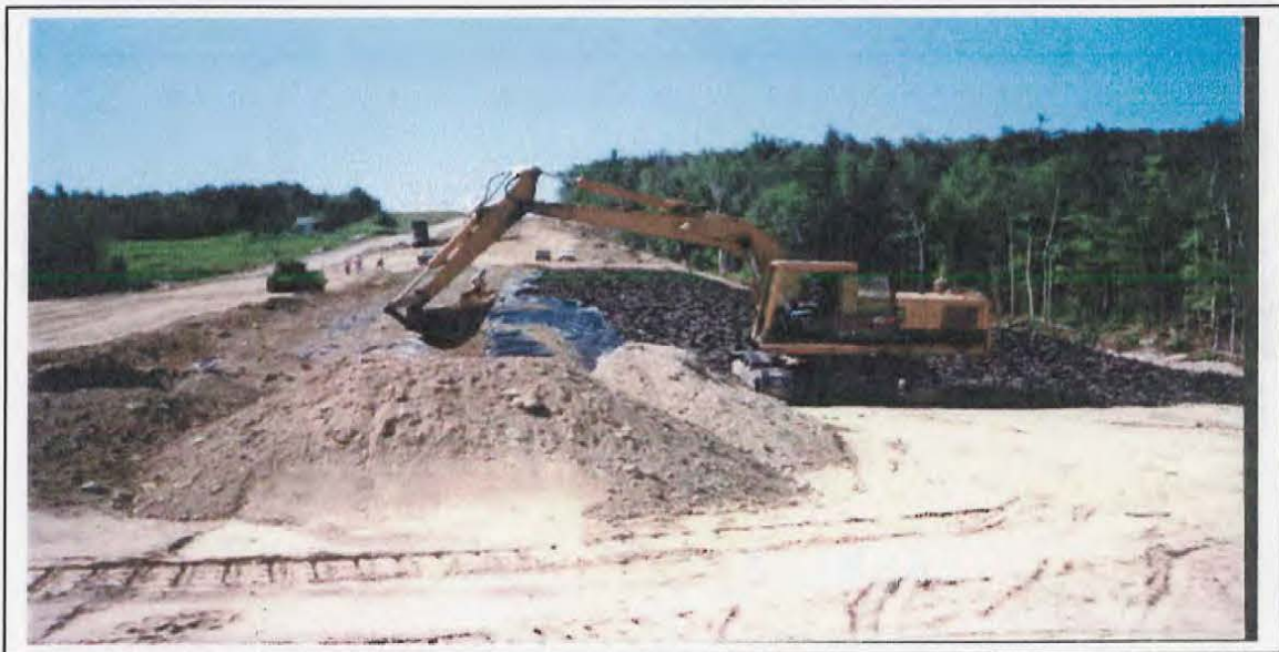
U.S. Route #9, Wesley, Me. road reconstruction project using type B modified tire chips as sub-base fill material
