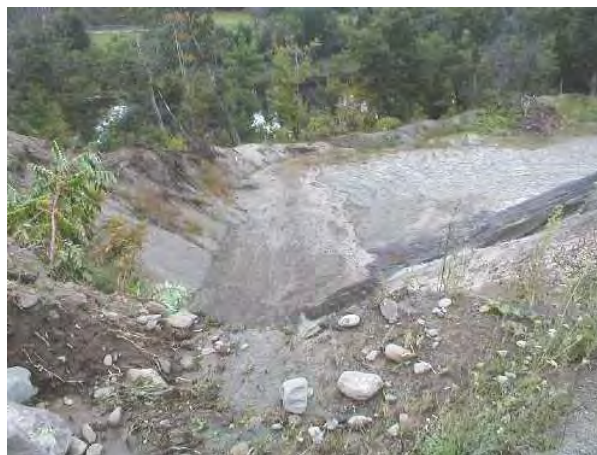
Figure 2. Ponding & infiltration on a steep slope.
