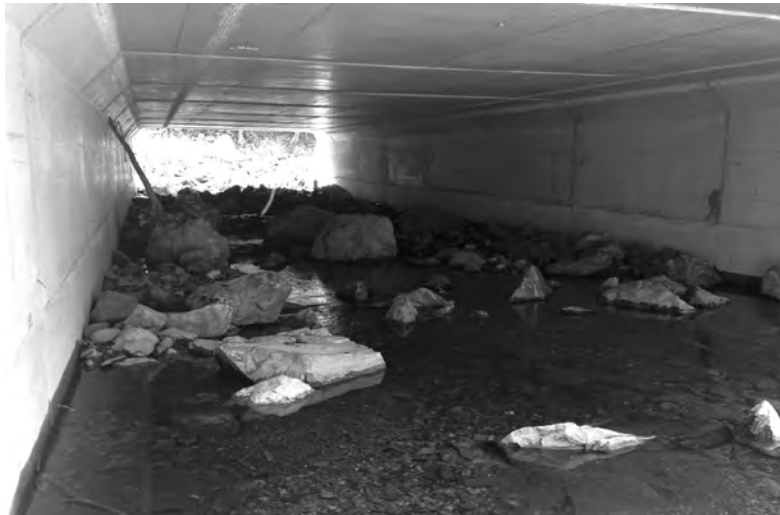
A box culvert. (Photo by MDIFW)
