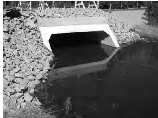
Figure 11. The upstream side of the same crossing after replacement. Photo Credit: Merry Gallagher.
