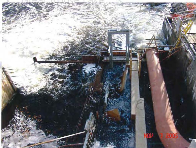
Flood at Burnham Fishway
