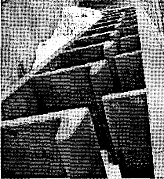
Figure 14. The lower sections of the fishway leading up to the corner pool.
