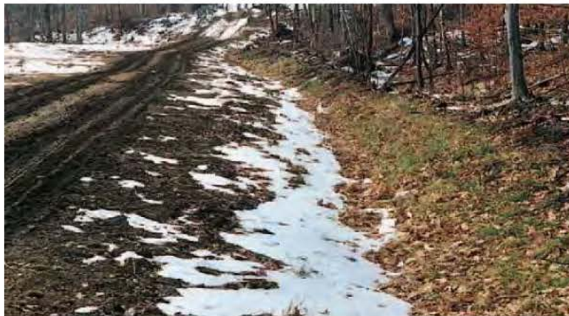
Revegetated road ditches carry water without eroding.
