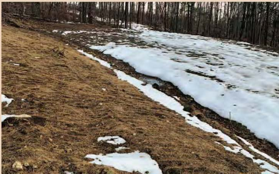
Hay mulch on landing.
