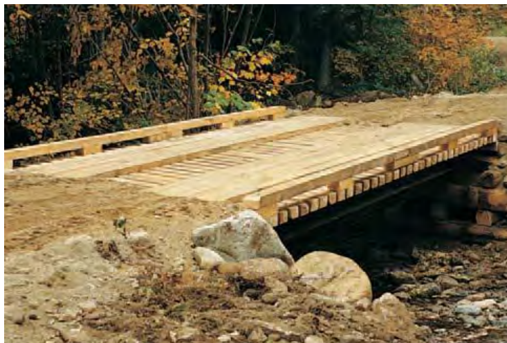
A permanent bridge.
