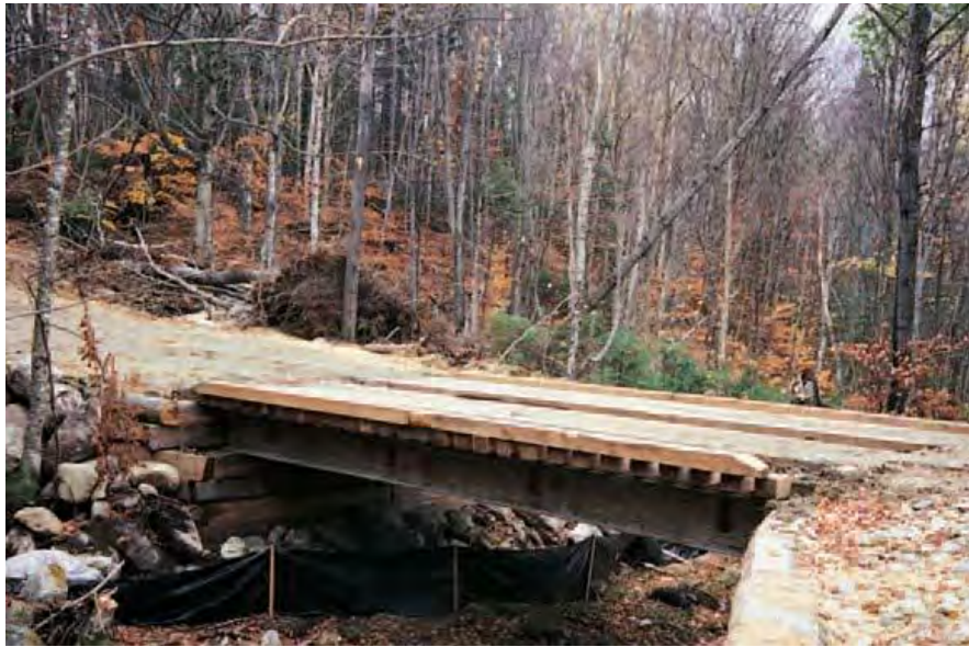
A permanent bridge on a truck road.
