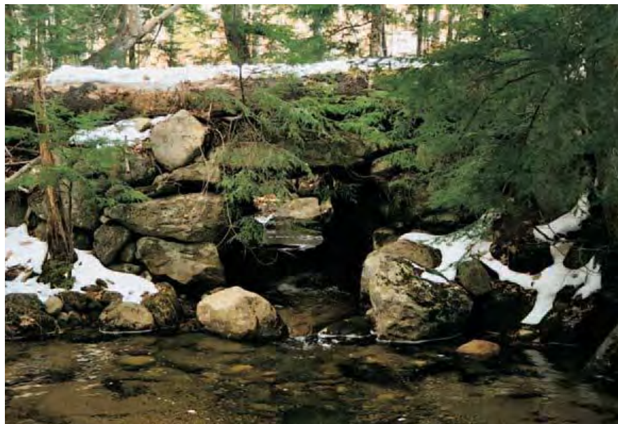
An old stone culvert still functioning.
