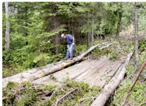
A temporary bridge.
