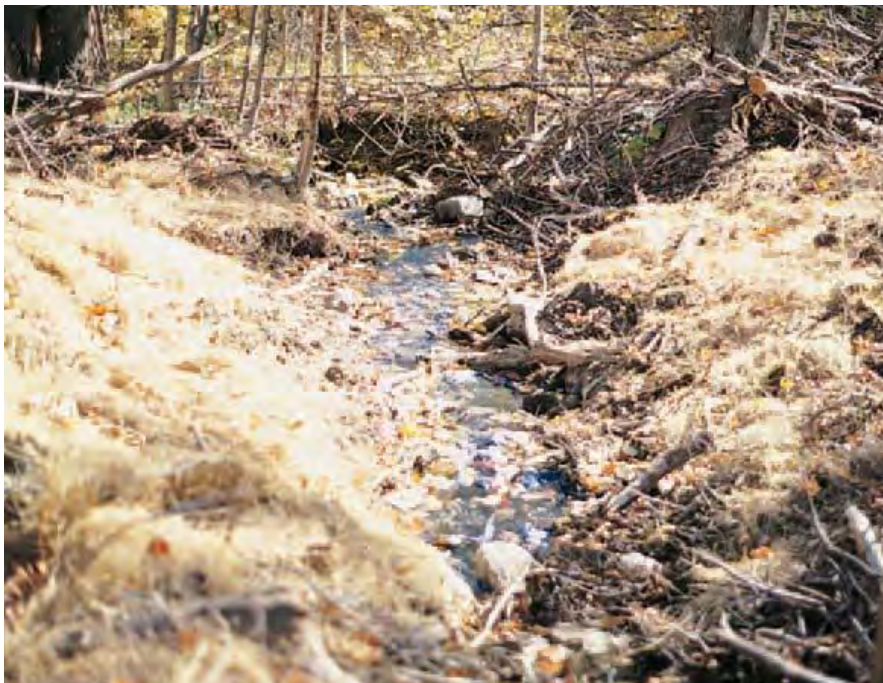
Closeout of a temporary stream crossing.
