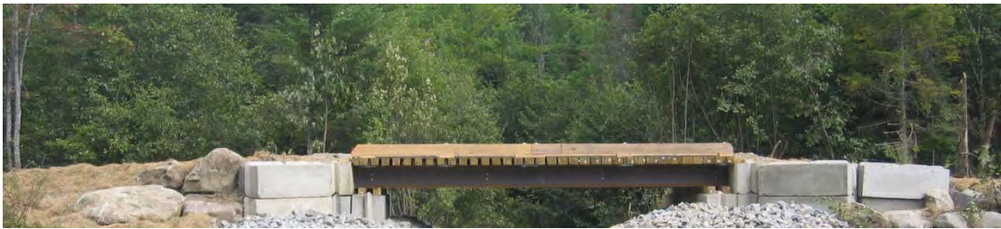
Note elevated crossing diverting water flow into filter areas
