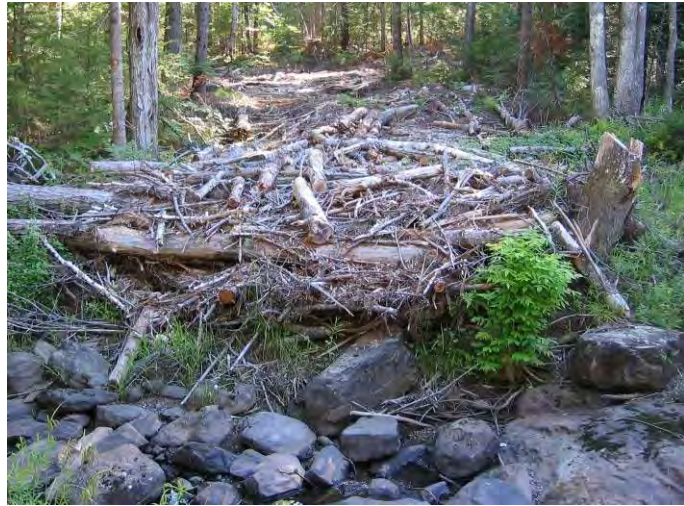
Well designed temporary crossings can be very cost effective and minimize disturbance to the waterbody. Pictured is the same crossing during use and after removal. Note that slash has been left on the approach to the crossing to stabilize any exposed soil. No sediment was deposited below the bankfull elevation of the channel.
