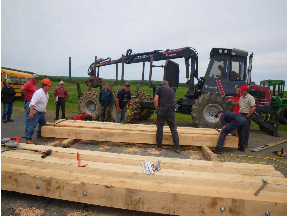
The Maine Forest Service and the Maine Sustainable Forestry Initiative sponsored skidder bridge mat workshops are designed to reduce stream crossing sedimentation by teaching loggers how to construct and install temporary skidder bridges. This program also provides direct assistance by providing skidder bridges that are available as free loaners at host mills.
