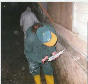
A new low-risk device for managing insect pests is installed on a Maine egg farm. A plastic sheet beetle barrier is attached with staples and latex caulk to walls and posts under a poultry barn.
