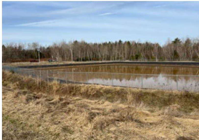
Leachate Lagoon at Pumpstation at Dolby Landfill
