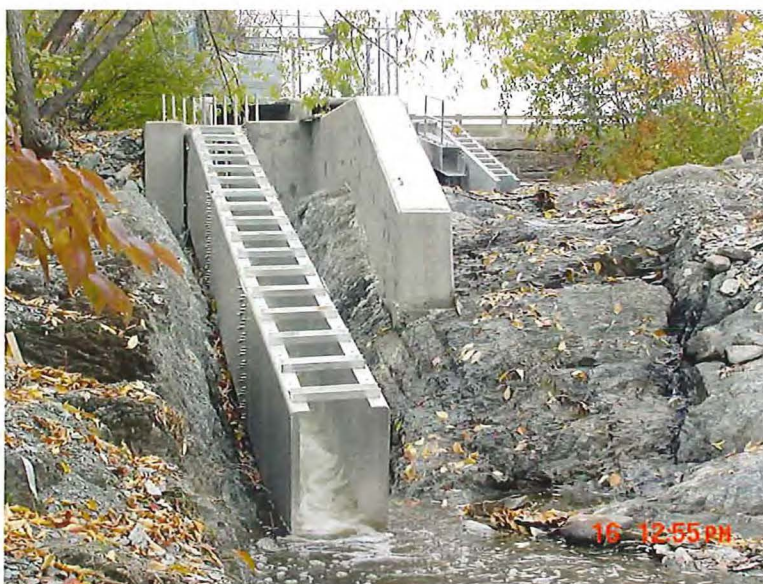
Figure 7. Alaskan Steeppass Fishways at Plymouth Pond Outlet Dam, October 2002
