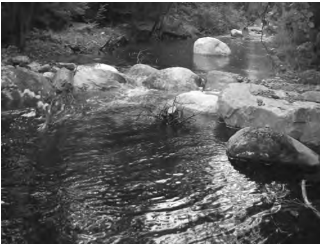
Figure 10. Rock weir with embedded root was constructed in 2007 showing scoured pool. Sandy River, Maine. Photo credit F. Bonney.
