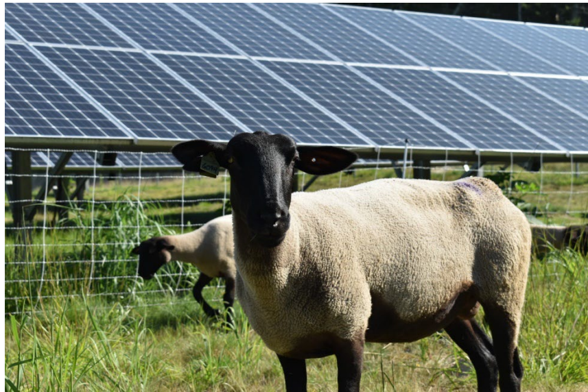
Photo credit: BlueWave Solar
