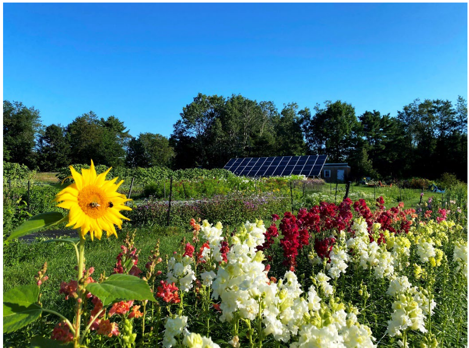
Photo credit: ReVision Energy
