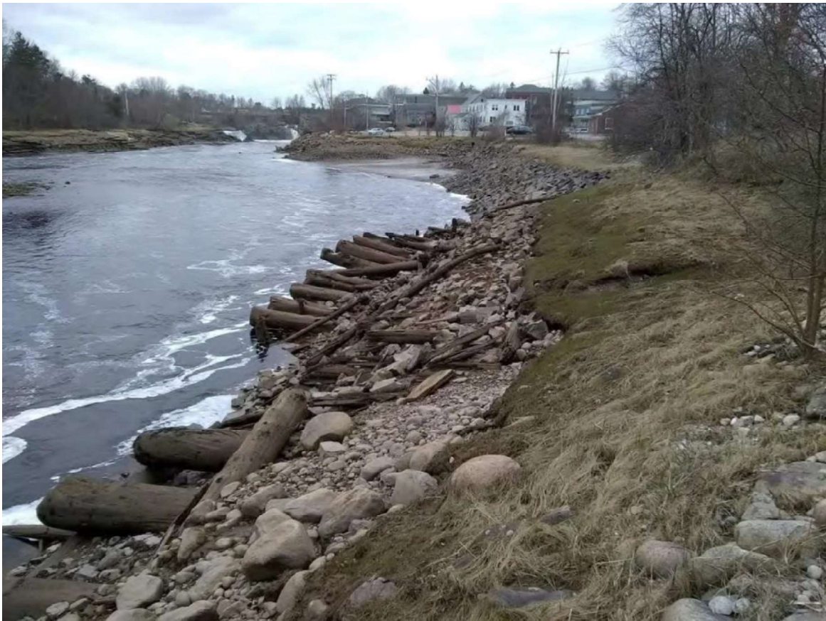
Figure 3 –2018 picture looking upstream with remnants of cribwork that supported former docks.
