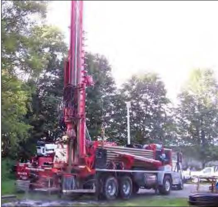
The first geothermal heating system in an executive branch facility being installed at the Department of Public Safety's State Police barracks in Skowhegan in 2009.
