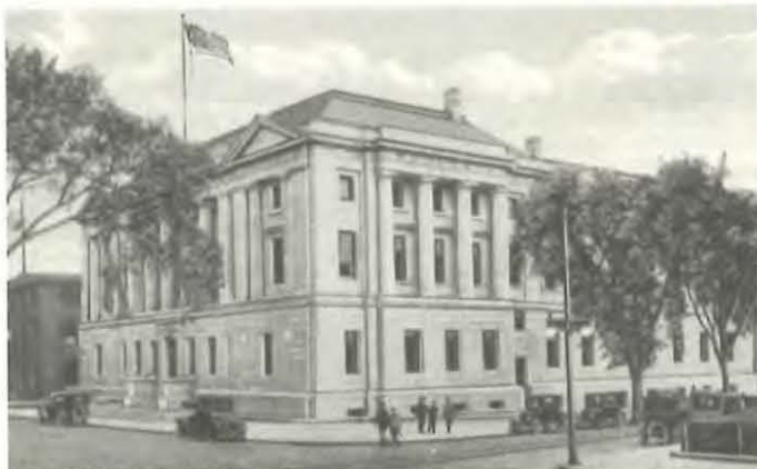
COUNTY COURT HOUSE, PORTLAND, MAINE
