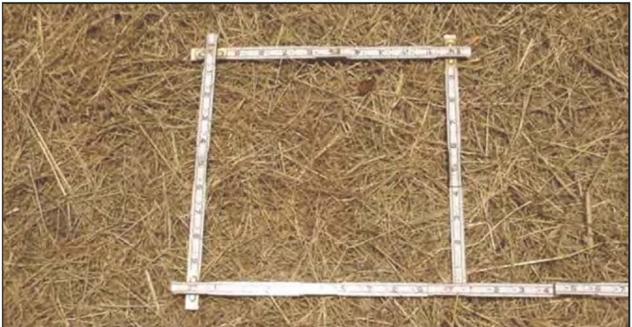
Figure 1. Hay Mulch - Adequate Application Rate
