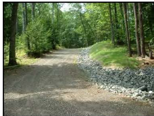
Same section of camp road several months after reconstruction.
