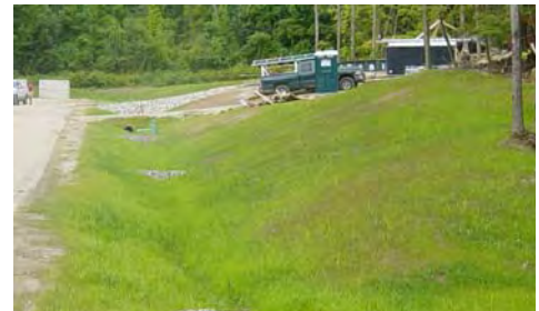
This ditch has been lined with grass to provide a permanent vegetative cover.
