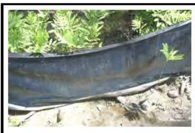
Pictured at left is an improperly installed silt fence. The bottom four inches of the fence should have been “keyed in,” such that a trench should have been dug out, the toe of the fence installed in the trench, and then backfilled.
