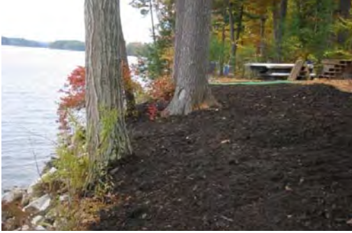
Erosion control mulch is applied here as a permanent mulch that will be a long-term cover to provide good buffer around a disturbed area.
