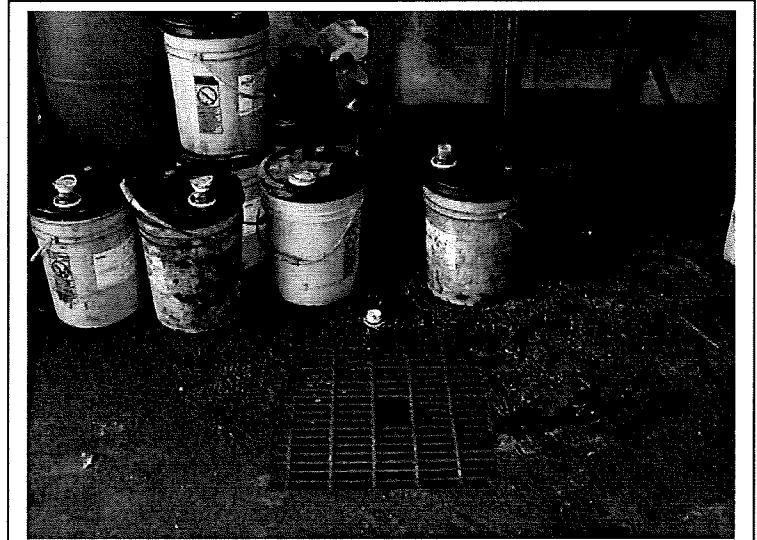
Oil and hazardous materials leaking into a floor drain
