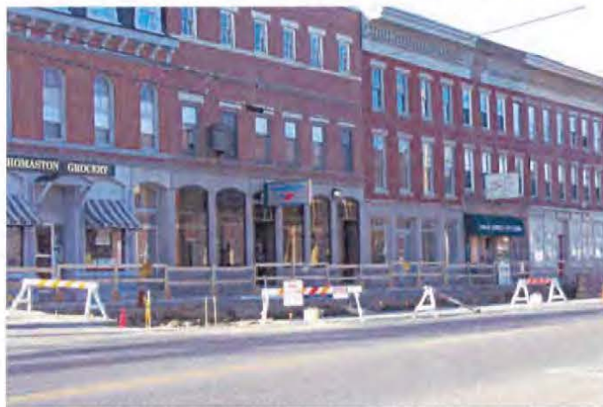
Downtown Thomaston, Sidewalk Project
