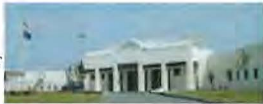
The new Maine State Prison - Warren February 2002
