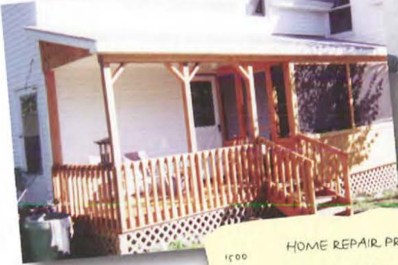
A MSHA FIX ME LOAN PROVIDES FUNDS NEEDED TO REPAIR THE PORCH ON THIS BANGOR HOME
