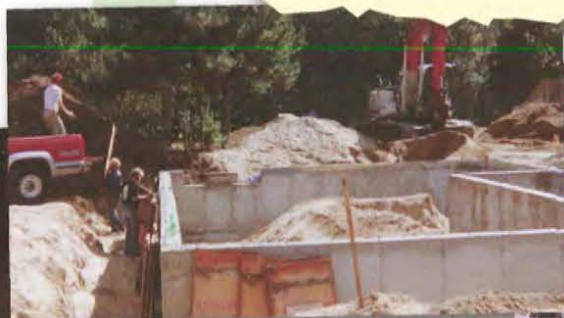
ONE OF FOUR FOUNDATIONS FOR A 12 UNIT RENTAL PROPERTY IN SOUTH PARIS
