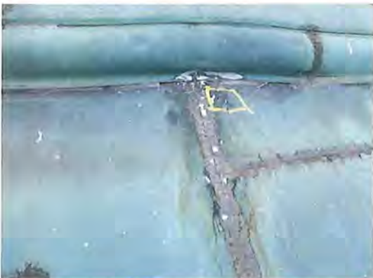
Open Holes at Copper At Upper Dome
