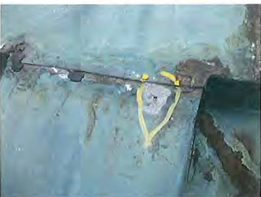
Open Holes at Copper At Upper Dome
