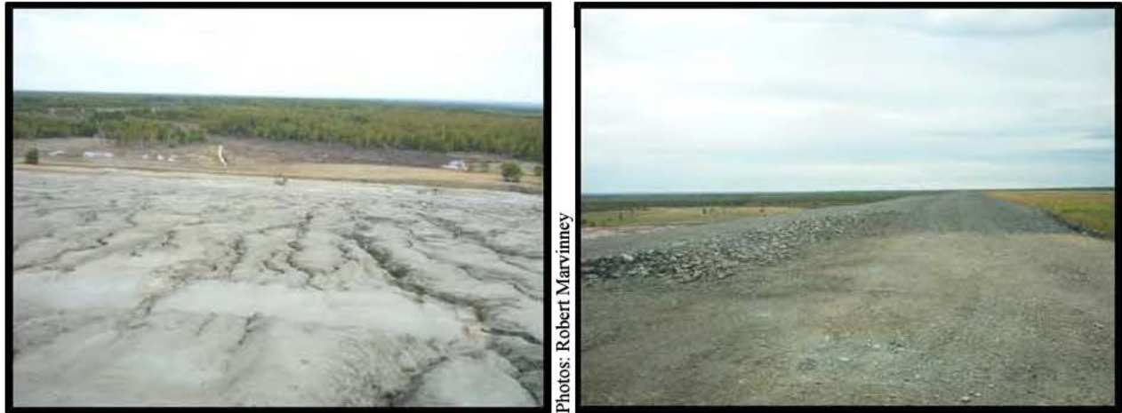
Tailings dam at a legacy mine. Left picture looks directly down the slope of the dam, built from tailings, showing significant gulley erosion. Right picture shows the top of the dam structure, with rock armoring along the left and stabilized tailings to the right. ( Brunswick No. 12 mine, New Brunswick. )
