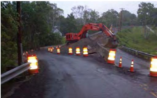
On June 16th, a teenager walking along **Route 24 in Harpswell** fell into a sinkhole adjacent to the road. Further investigation revealed that a 30-inch diameter, 106-foot long metal cross culvert had corroded and failed. By nightfall, a MaineDOT crew had filled the hole and barricaded the site. Plans were devised to immediately replace the pipe. The project was complex, since the pipe was 24 feet below the
